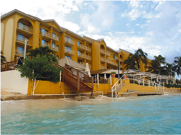
Fig. 13a. Marriott Beach Resort shoreline October 2012. Note the wooden steps onto the beach which indicate long-term reduction in beach volume.
