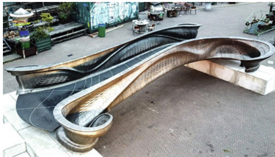
Fig. 16 Metal footpath bridge from the Dutch Design Week 2018 [61]. Reprinted from Journal of Constructional Steel Research. 172, Gardner, L., Kyvelou, P., Herbert, G., Buchanan, C.: Testing and initial verification of the world’s first metal 3D printed bridge, 106,233 (2020), with permission from Elsevier
