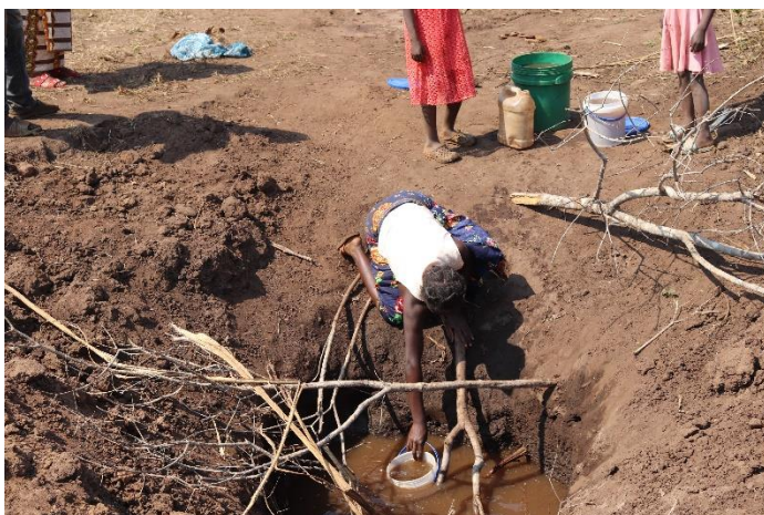
Figure 4: Scoop holes dug in the stream or river beds to access water during the dry seasons
