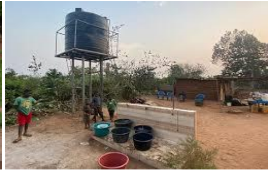
Picture 2: Borehole overhead storage
