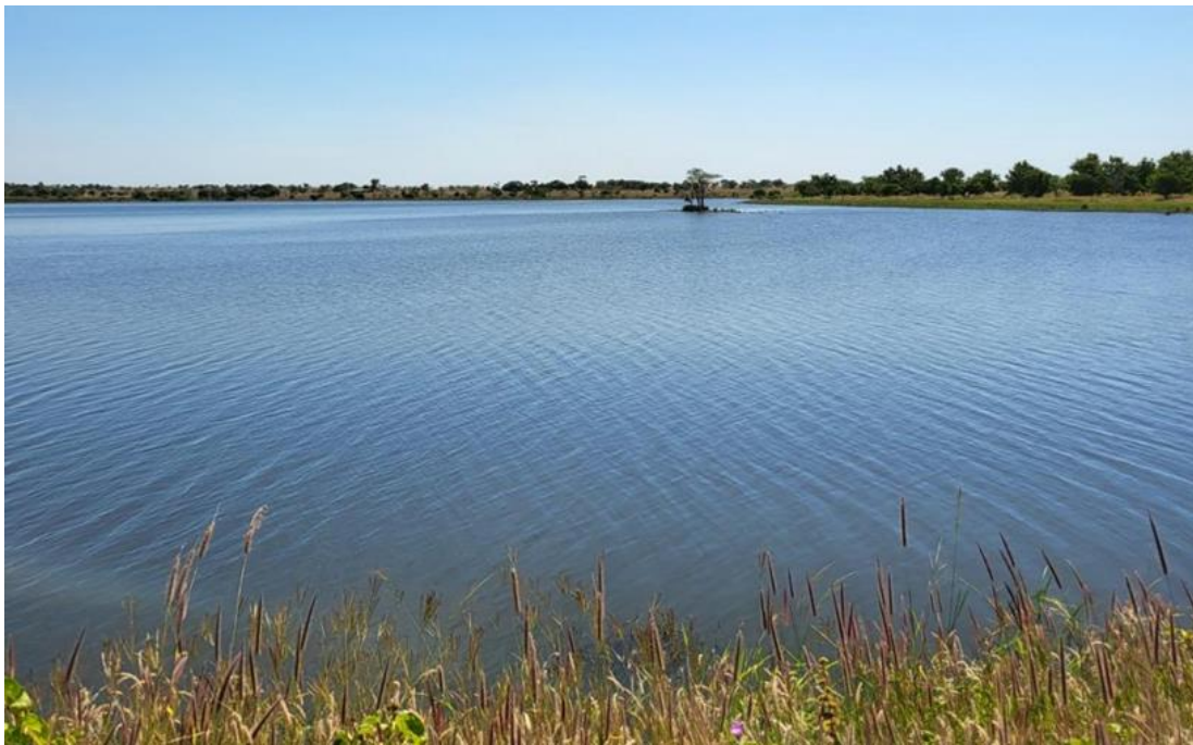
Figure 8. A picture of the Nansoni dam.
