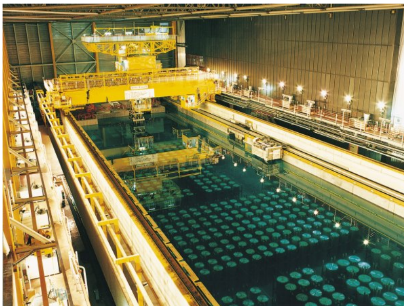
FIGURE 1.3. Storage pond at the UK's Sellafield for the used fuel. Figure from [20].
