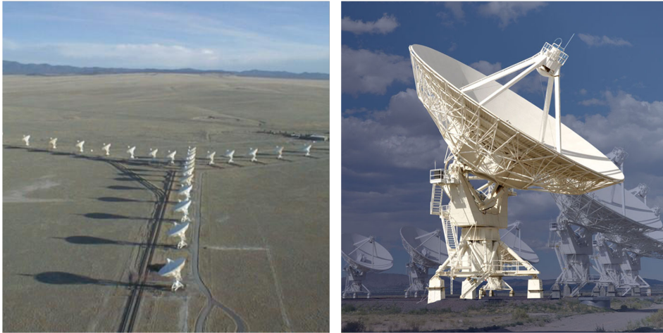
Figure 2.3: Left: Overall view of the VLA, looking south in a compact configuration. The array can be reconfigured by moving the antennas to more distant pads via the rail lines visible in the photograph. Right: A close-up image of one of the 25 m diameter antennas in the array – (Credit: Dave Finley, NRAO/AUI).
