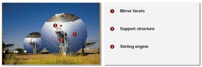
Figure 2-5: The PDS main components [49].
