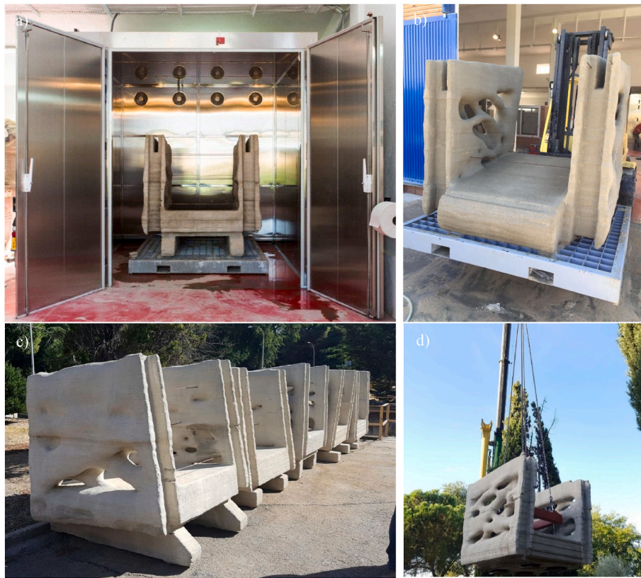
Fig. 3. (a) Accelerated curing chamber, b) transport of a segment to the external yard, a) segments stored at yard environmental conditions, and d) 4-point lifting of the segments with a single crane.
