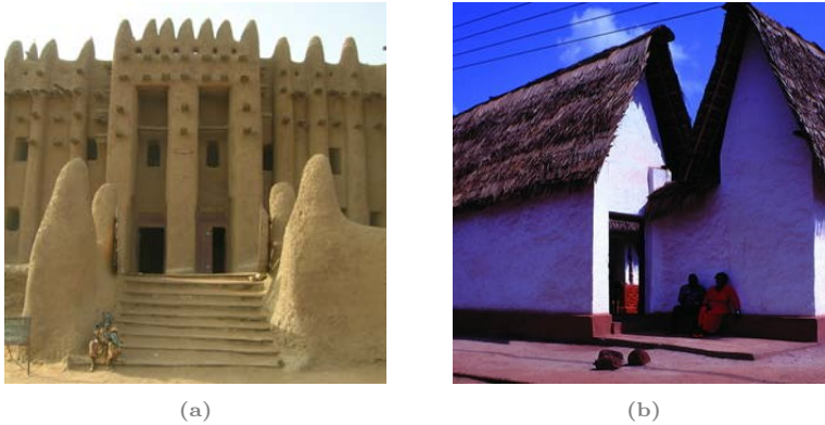
Figure 2.3: Earth construction in Africa: (a) Old Town of Djenné, Mali (©F. Bandarin, UNESCO) and (b) traditional earth house in Asante, Ghana (©T. Joffroy, CRA-terre).
