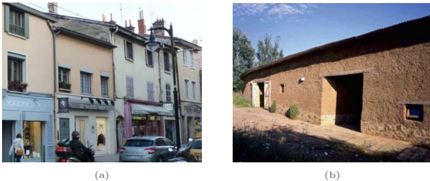
Figure 2.10: Monolithic earth constructions: (a) rammed earth dwellings in Lyon, France [24] and (b) cob house in Worcester, UK [13]
