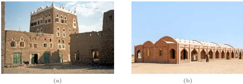
Figure 2.7: Earth block construction: (a) adobe building in Sa'dah, Yemen (©B. Gagnon, Wikimedia Commons) and (b) Primary School Tanouan Ibi, Mali, made of CEB (©Levs Architecten).
