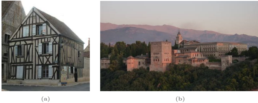
Figure 2.4: Earth construction in Europe: (a) wattle and daub house in the medieval town of Provins, France (©E. Westerveld) and (b) the Alhambra of Granada, Spain (©P. Schinz).
