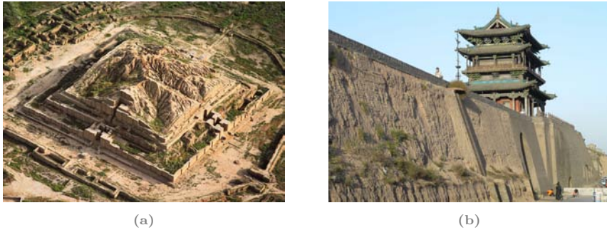
Figure 2.2: Historic earth constructions in Asia: (a) Chogha Zanbil ziggurat, Iran (©G. Gerster, AGE Fotostock) and (b) rammed earth wall of the Ancient City of Ping Yao, China (©T. Joffroy, CRA-terre).
