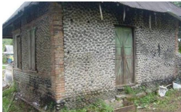
Figure 2.2 Example of URM building classified as MUR+STRUB/LWAL/H:1 according to [42]
