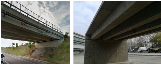
Fig. 1 The existing bridge (on the left) and the investigated scaled model (on the right)
