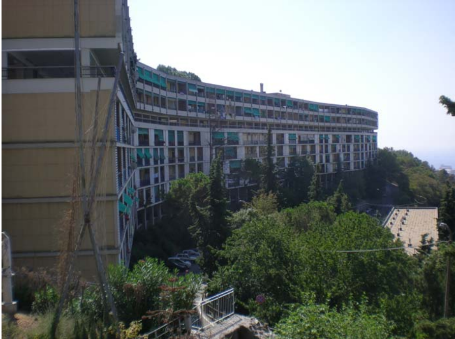
Fig. 3 - The relationship between the Biscione's building E and the surrounding green spaces
