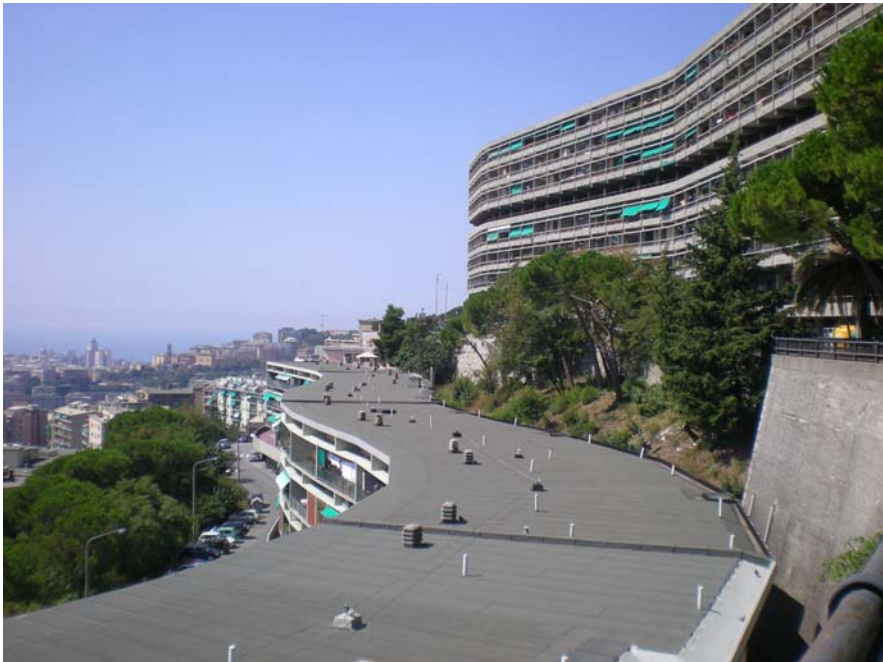
Fig. 2 - A panoramic view of the Biscione’s building A towards the city centre and the sea
