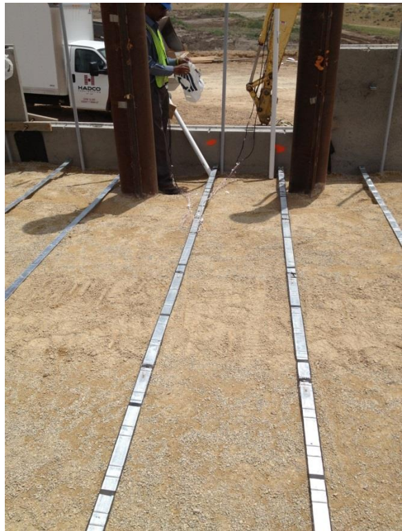
Figure 4.2: Photographs of reinforcement installation.
