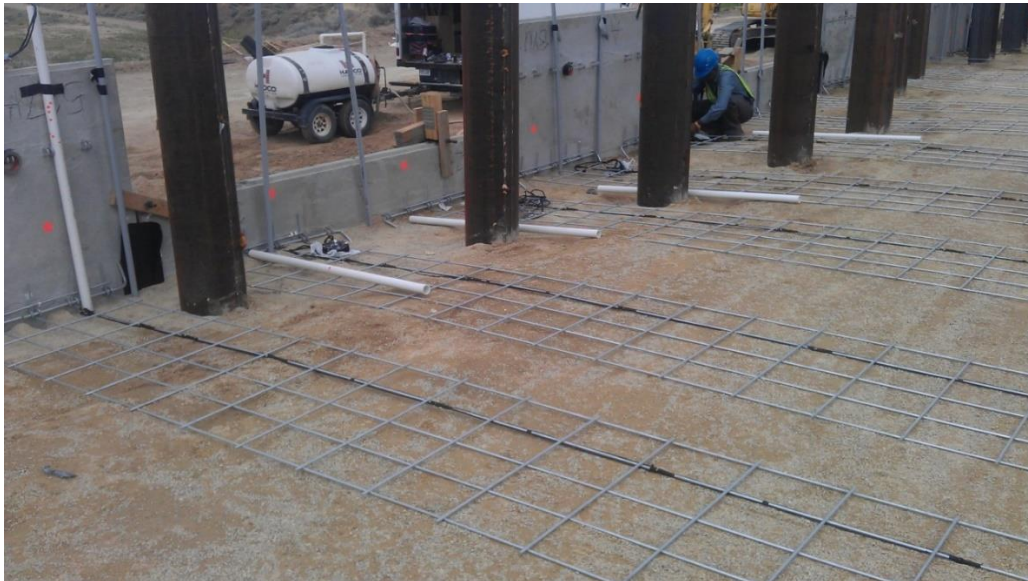
Figure 4.6 Instrumented grids being placed in the fill.
