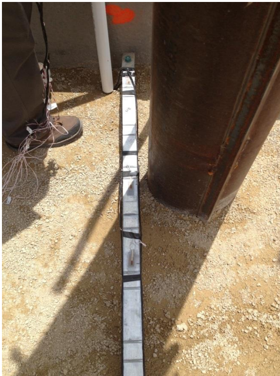
Figure 4.2: Photographs of reinforcement installation.
