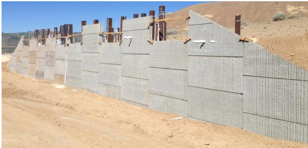
Figure 5.1: Photograph of the MSE wall at the time of testing.
