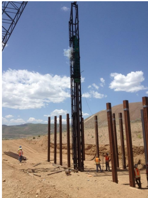
Figure 3.14: Pile driving using a diesel hammer.
