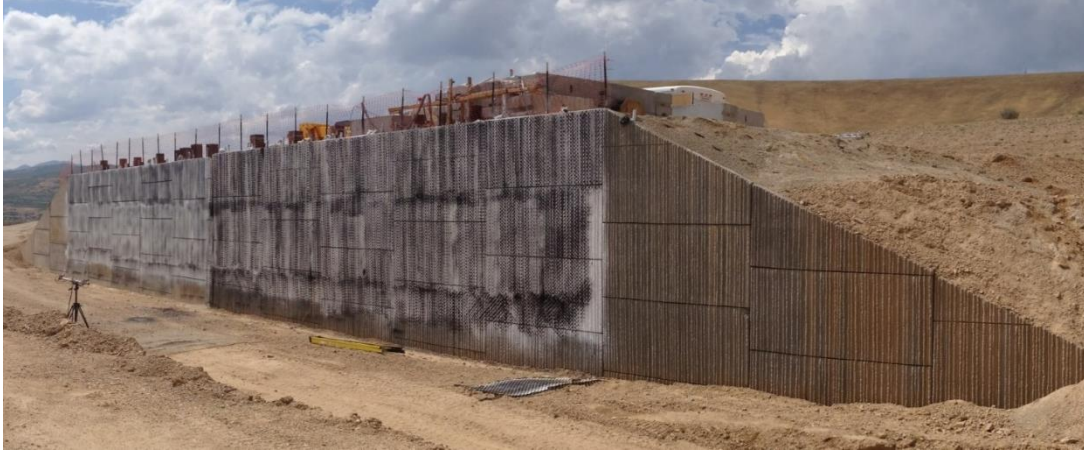
Figure 6.1 Photo of the wall at the time of testing.
