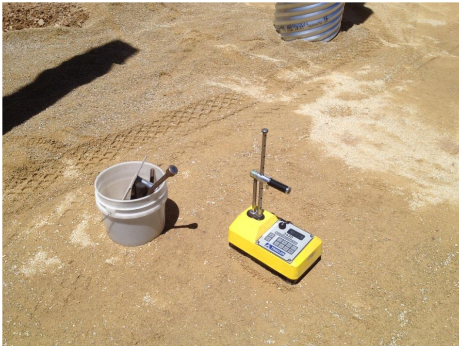
Figure 3.11: In-place nuclear density gauge test.
