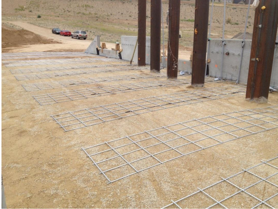
Figure 3.7: Welded wire grid reinforcements.
