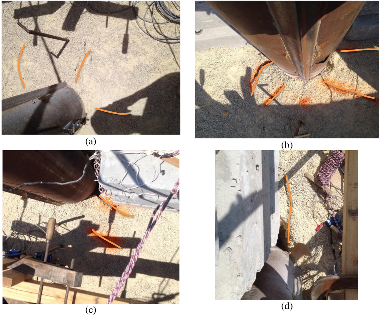
Figure 6.21 Cracks in the ground surface testing, (a) 5.3D (b) 4.3D (c) 3.2D (d) 1.9D.
