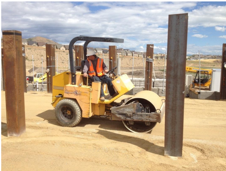
Figure 3.9: Roller compaction between test and reaction piles.
