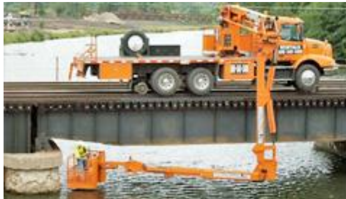
Figure 6: Under Bridge Inspection Vehicle
