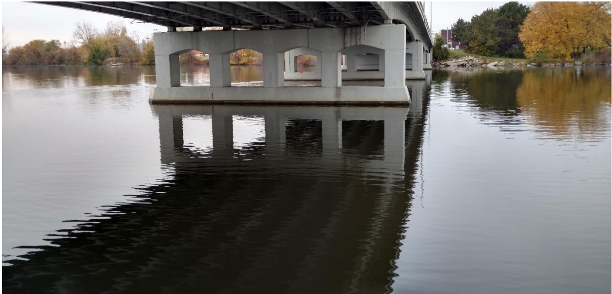
The above photo shows the western channel bridge is a single pile cap with four concrete columns reaching upward to support a single top header beam. With just the 2-inch tall antenna, the EMILY LOS kept disconnecting from the shore station, so at 0830 hrs the 4 foot antenna was attached and is slightly visible just over the pier wall in the photo below.
