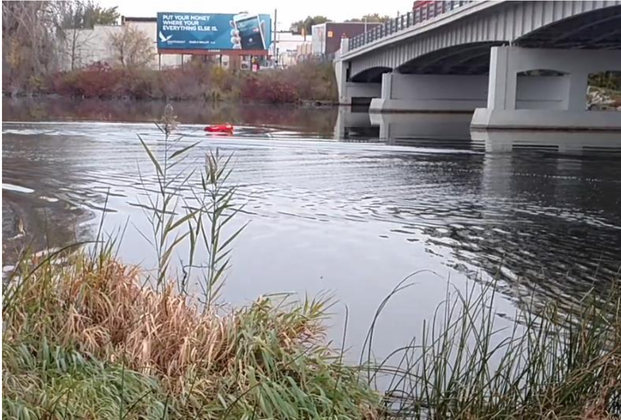
The above photo shows the western channel bridge is a single pile cap with four concrete columns reaching upward to support a single top header beam. With just the 2-inch tall antenna, the EMILY LOS kept disconnecting from the shore station, so at 0830 hrs the 4 foot antenna was attached and is slightly visible just over the pier wall in the photo below.
