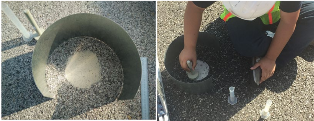
Figure 1.4 SPT equipment (left), and field data collection (right)
