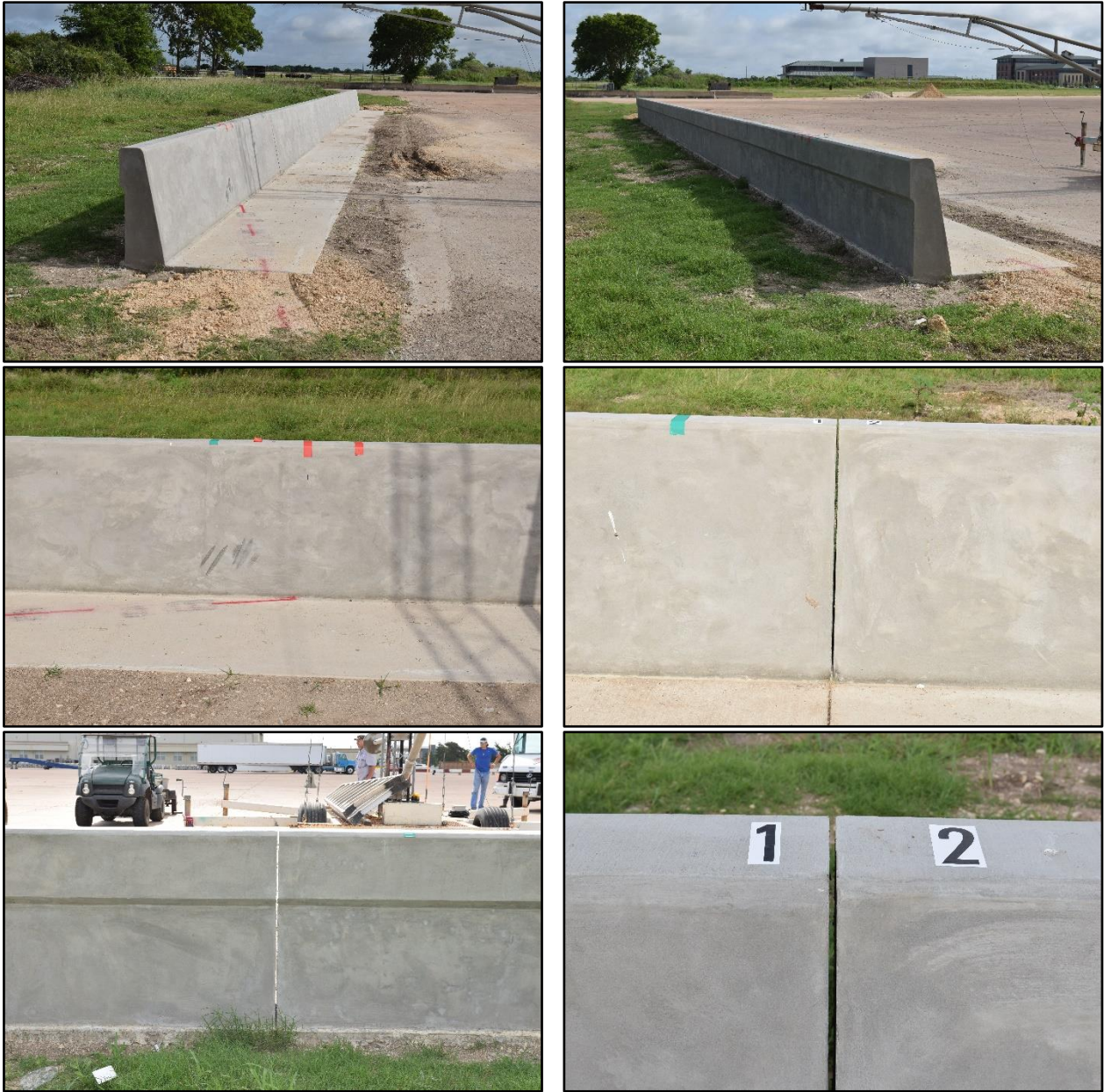
Figure 3.2. SSTR with Moment Slab Foundation Prior to Testing.
