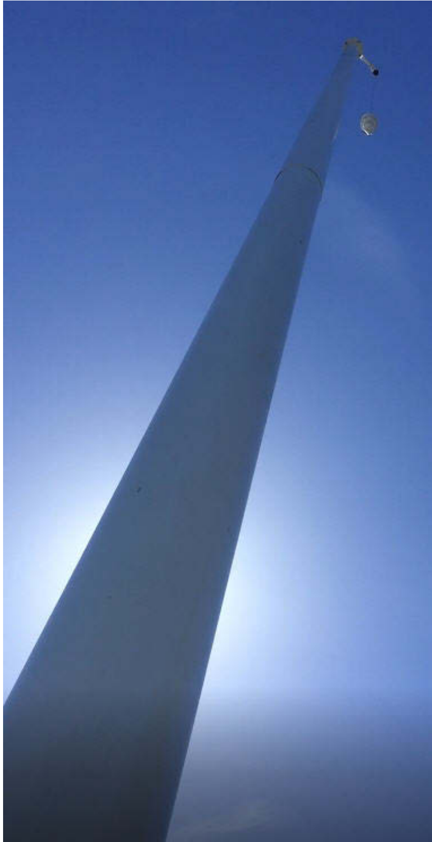
Figure 20. Bay Bridge High-Mast MG 2 Internal-Type CLD System
