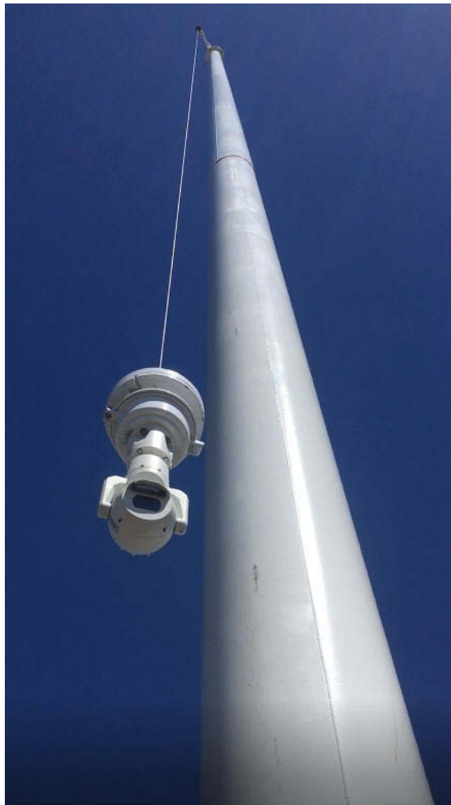
Figure 64. Bay Bridge MG 2 Internal-Type CLD
