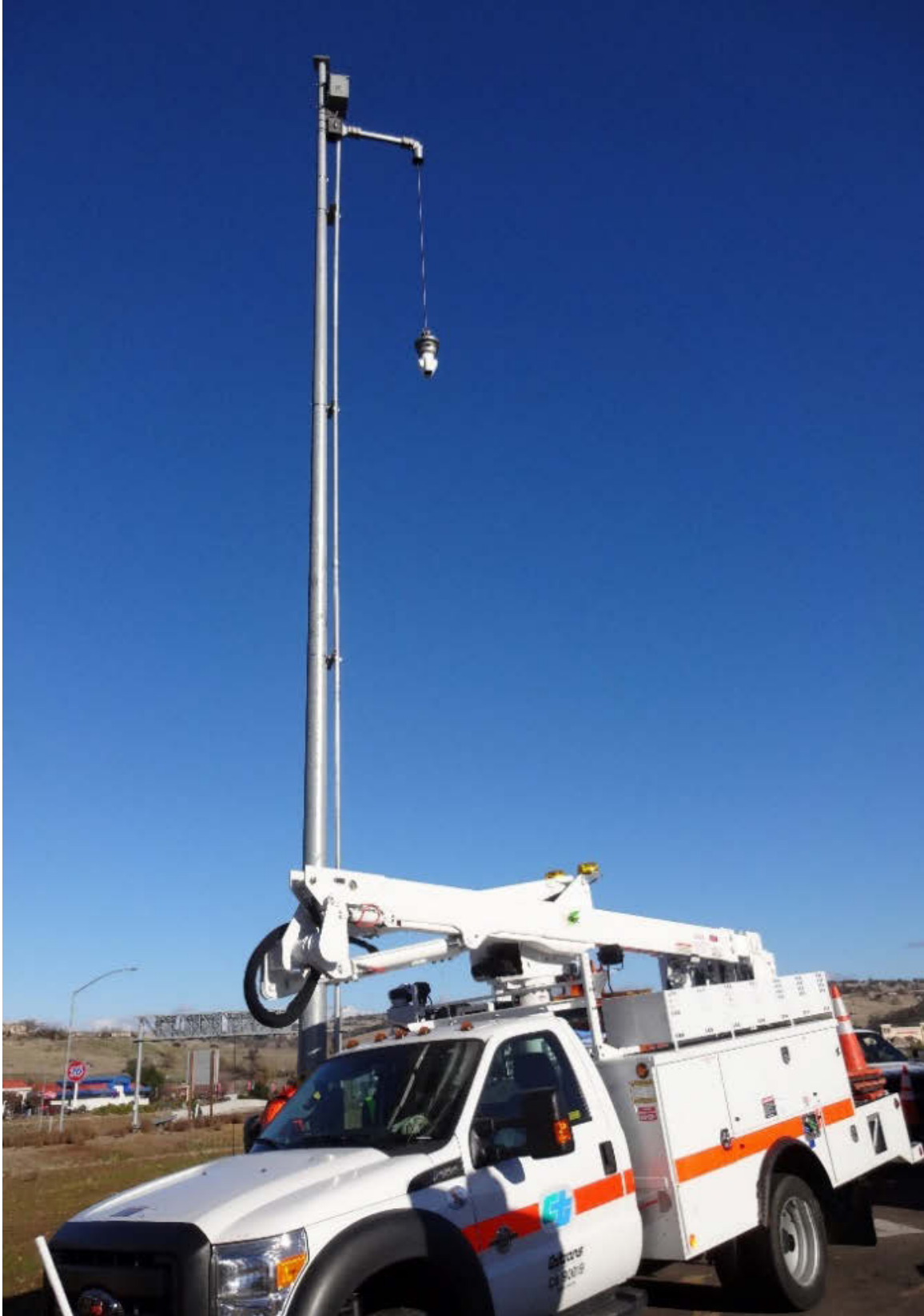
Figure 46. Lowering CCTV Camera MG2 External-Type CLD
