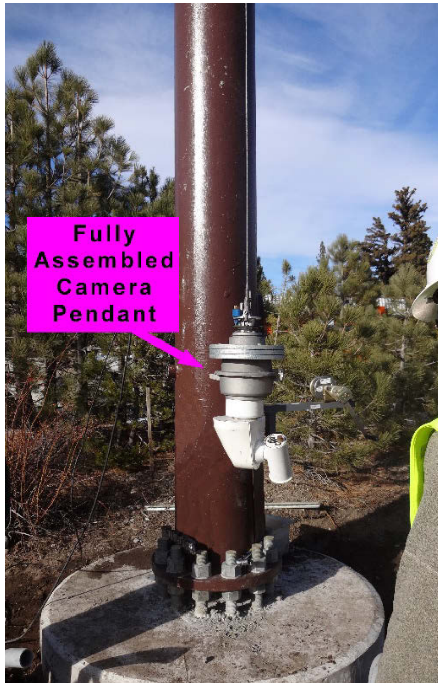
Figure 38. Fully-Assembled Camera, Pendant Lowered
