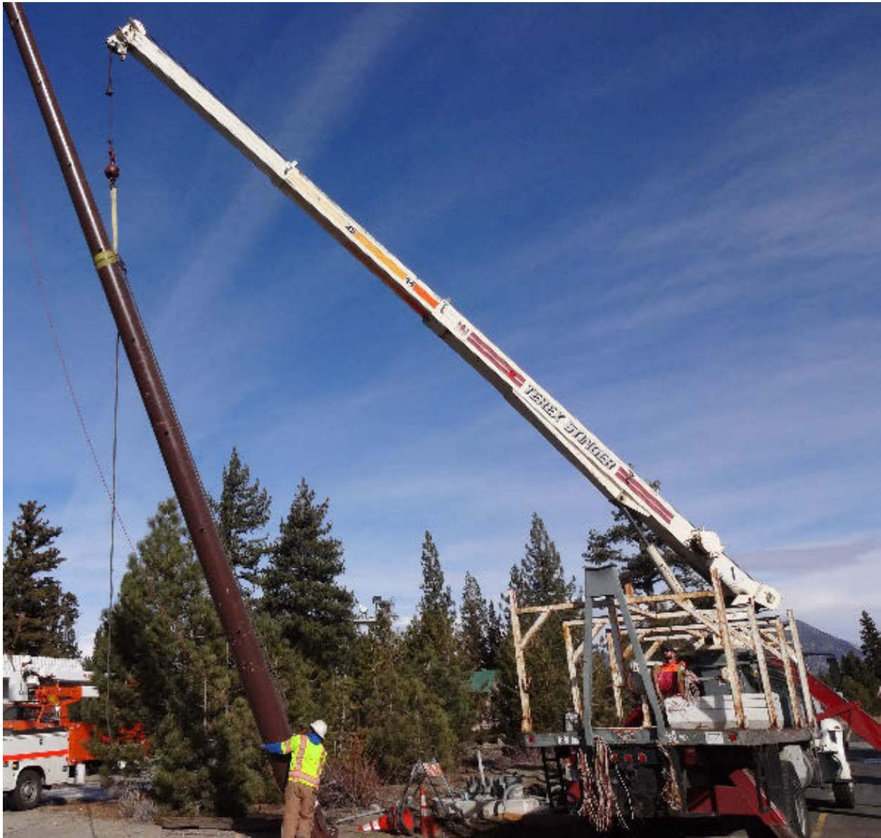
Figure 29. Crane Truck Erecting Pole
