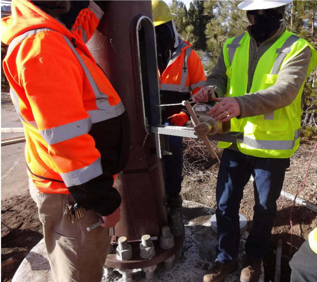
Figure 34. MG 2 CLD Winch Tool Attached
