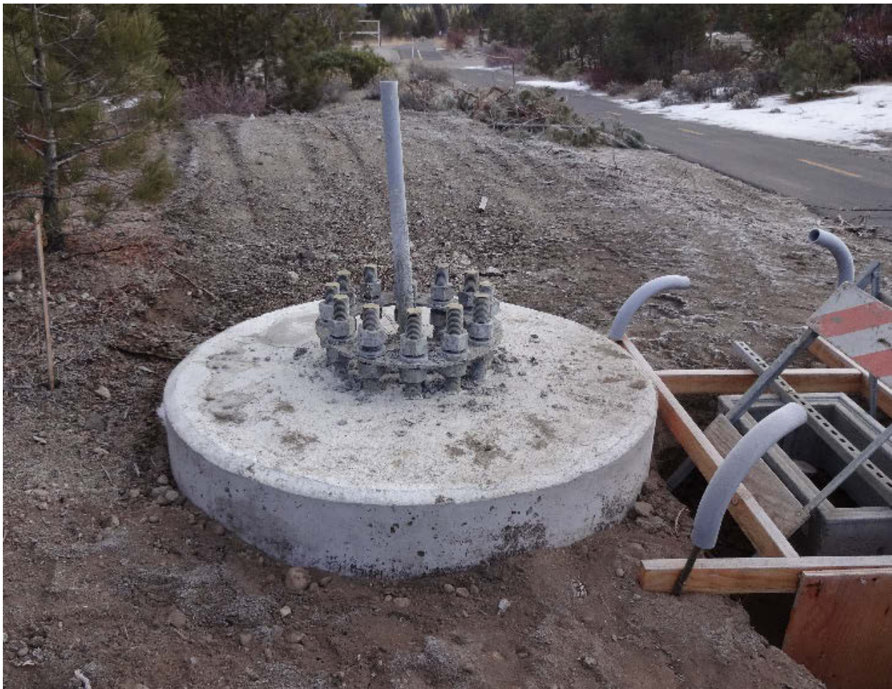
Figure 28. MG 2 Internal-type CLD Pole Footing
