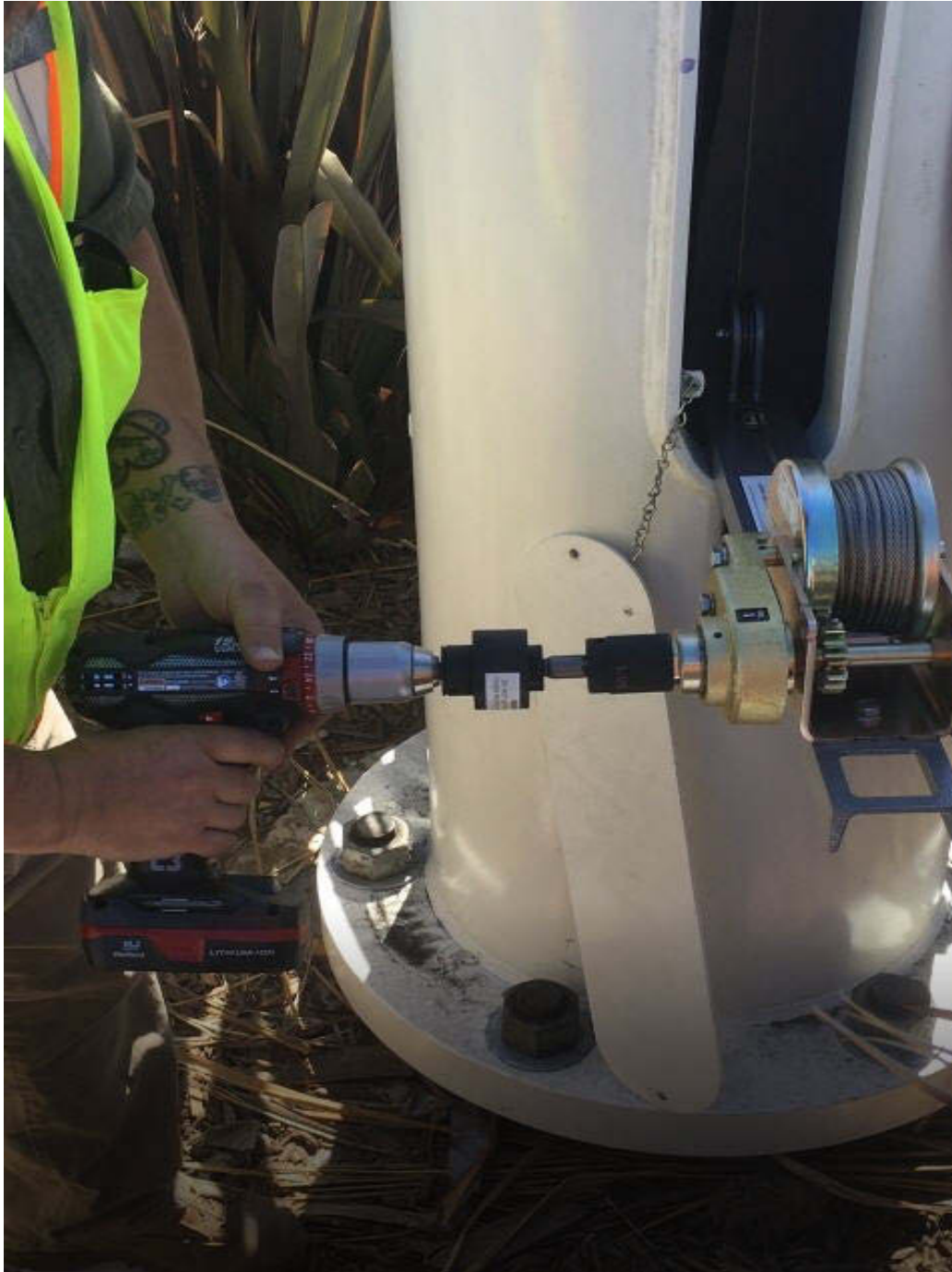
Figure 5. MG 2 Portable Winch Tool and Handheld Drill Motor Driver
