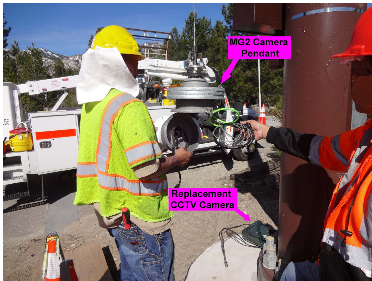
Figure 52. CCTV Camera Replacement
