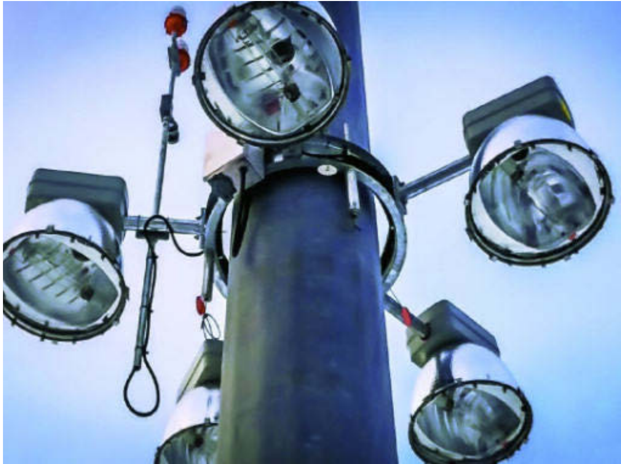
Figure 21. Halo High-Mast Lighting Application
