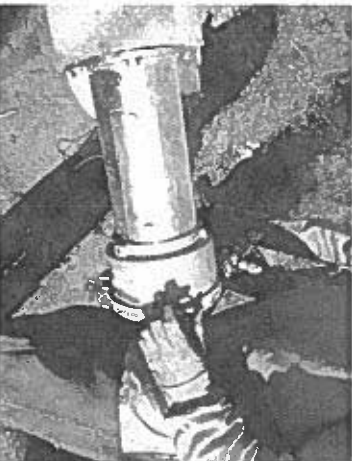
Secure the Pole-Top Junction Box and cover.
