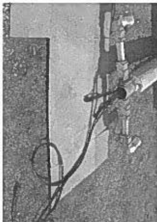
Feed Power/Signal Cable Down Pole
