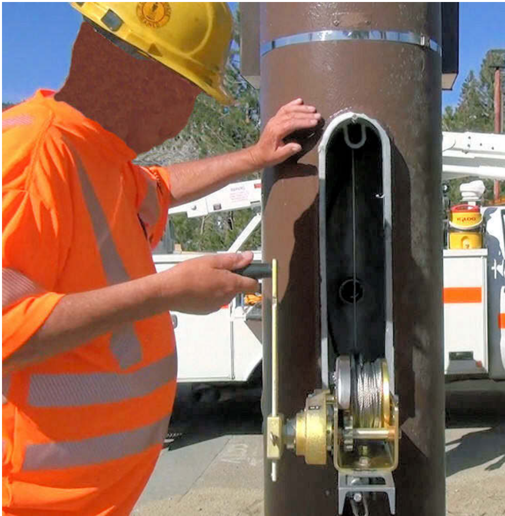
Figure 51. Hand Cranking Winch
