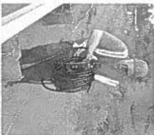
Unroll Composite Cable Hand over Hand to avoid Kinks
