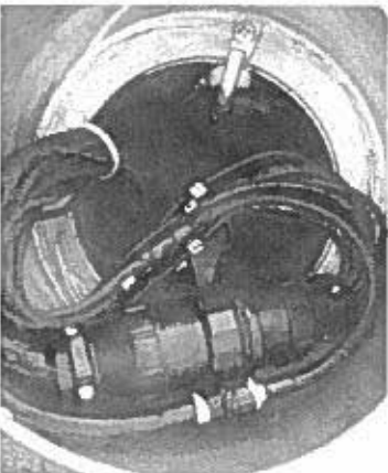
Secure Power/Signal Cable inside Pole Top Junction Box
