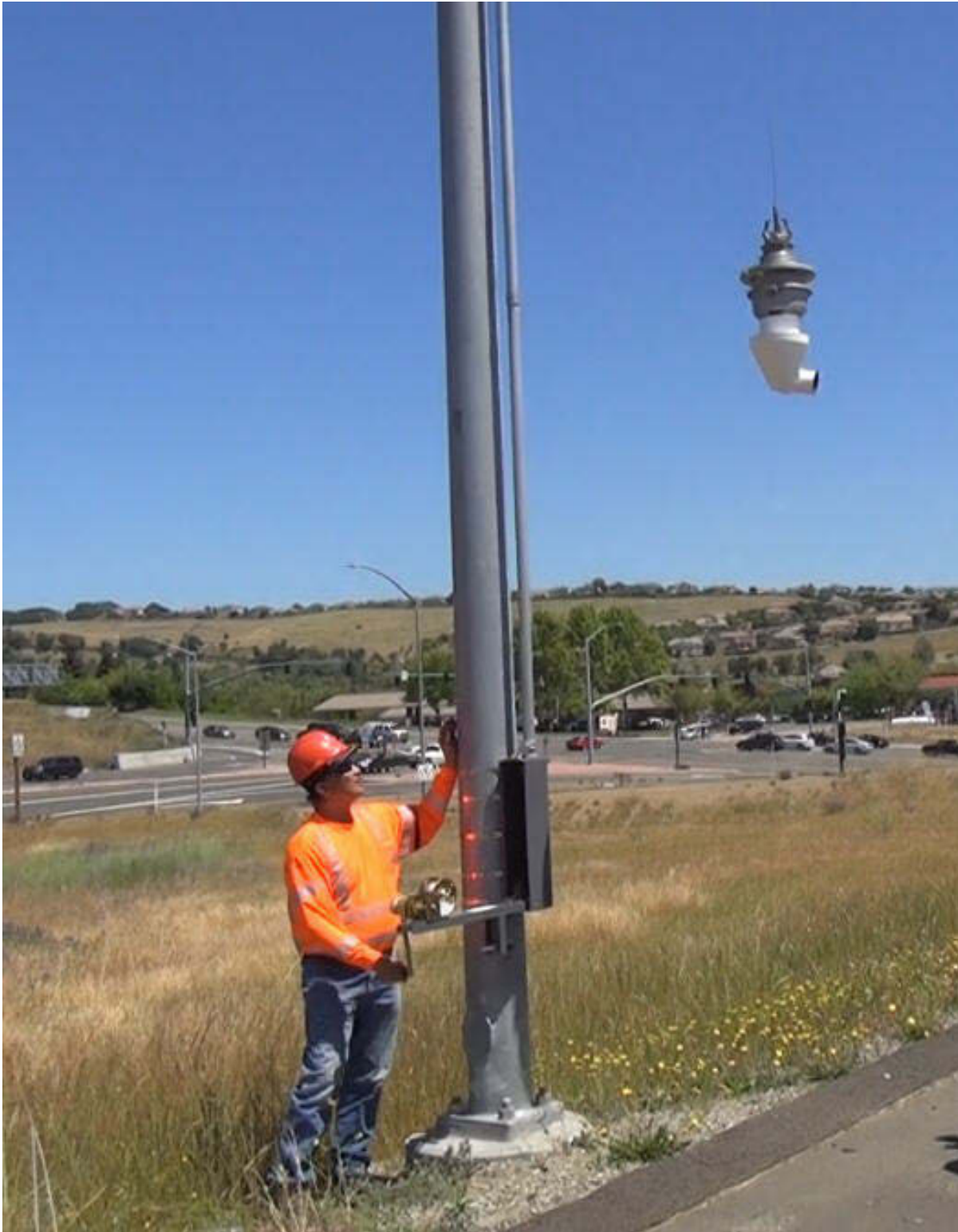
Figure 57. MG 2 External-Type Camera Lowering
