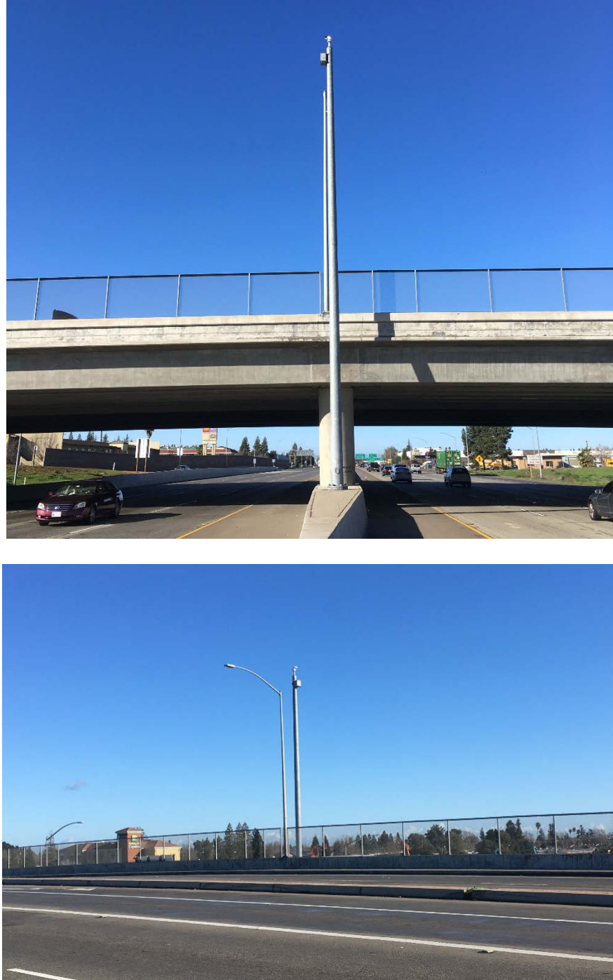
Figure 1. High-Mast Fixed Camera Mounting with Overpass Access
