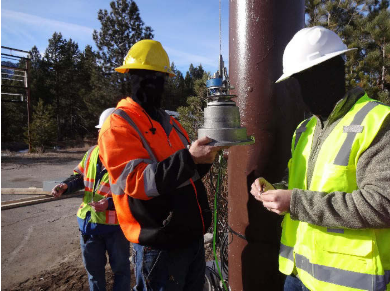
Figure 36. Attaching Coupling Junction Box
