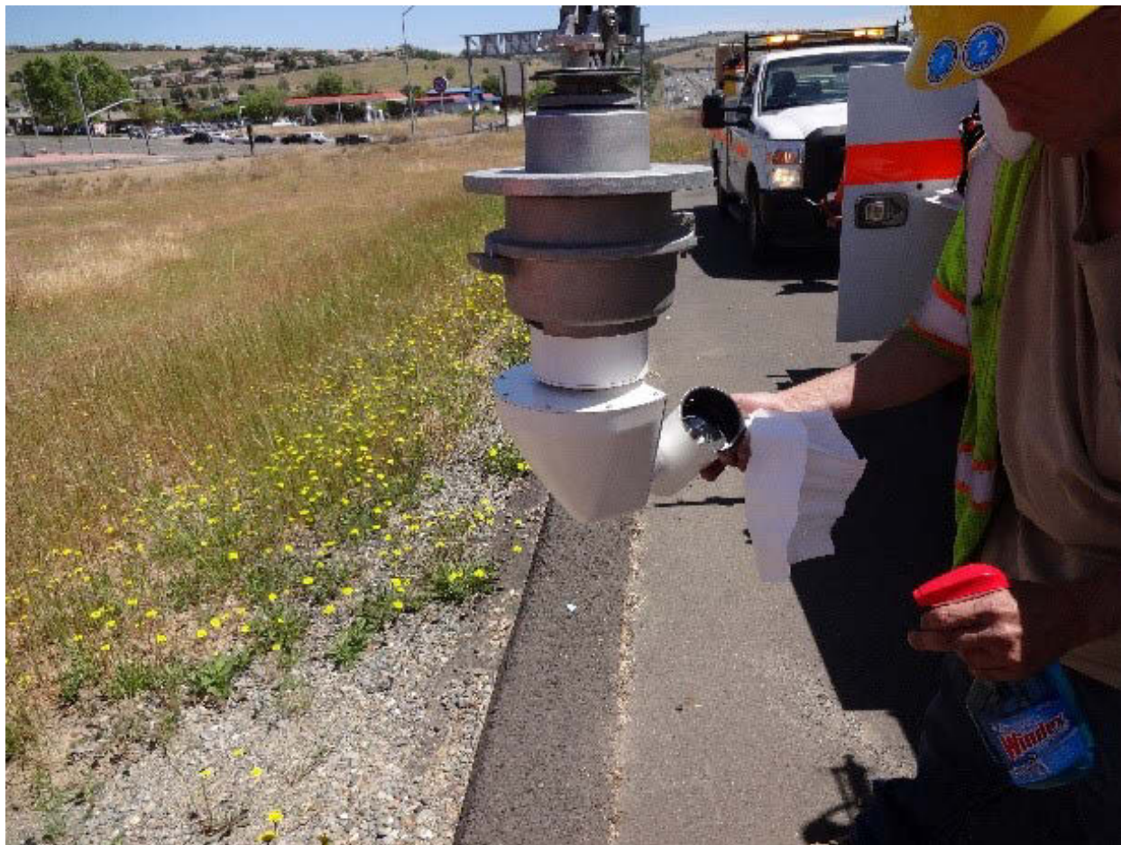
Figure 58. CCTV Lens Cleaning
