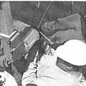
Keeping slight tension on the Lowering cable, engage the bottom contact and perform a continuity check
