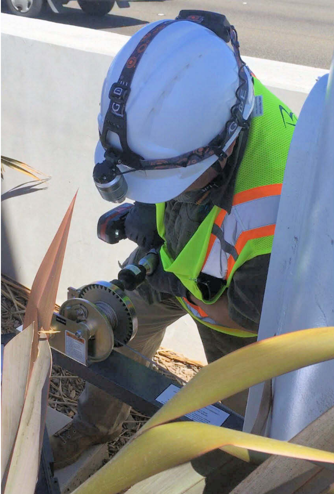
Figure 61. Power Driving Winch Tool
