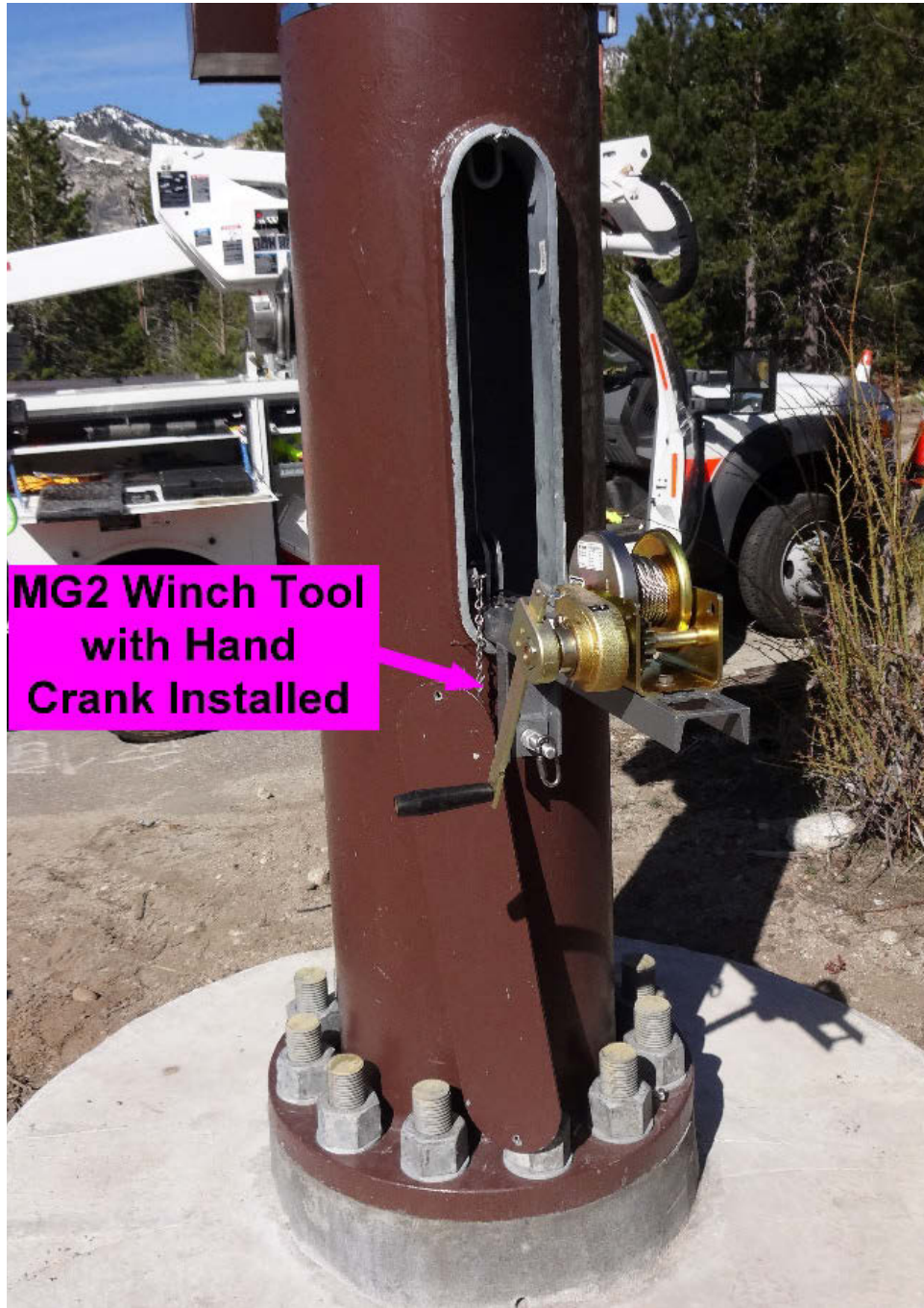
Figure 49. Meyers MG 2 Lowering Winch Tool
