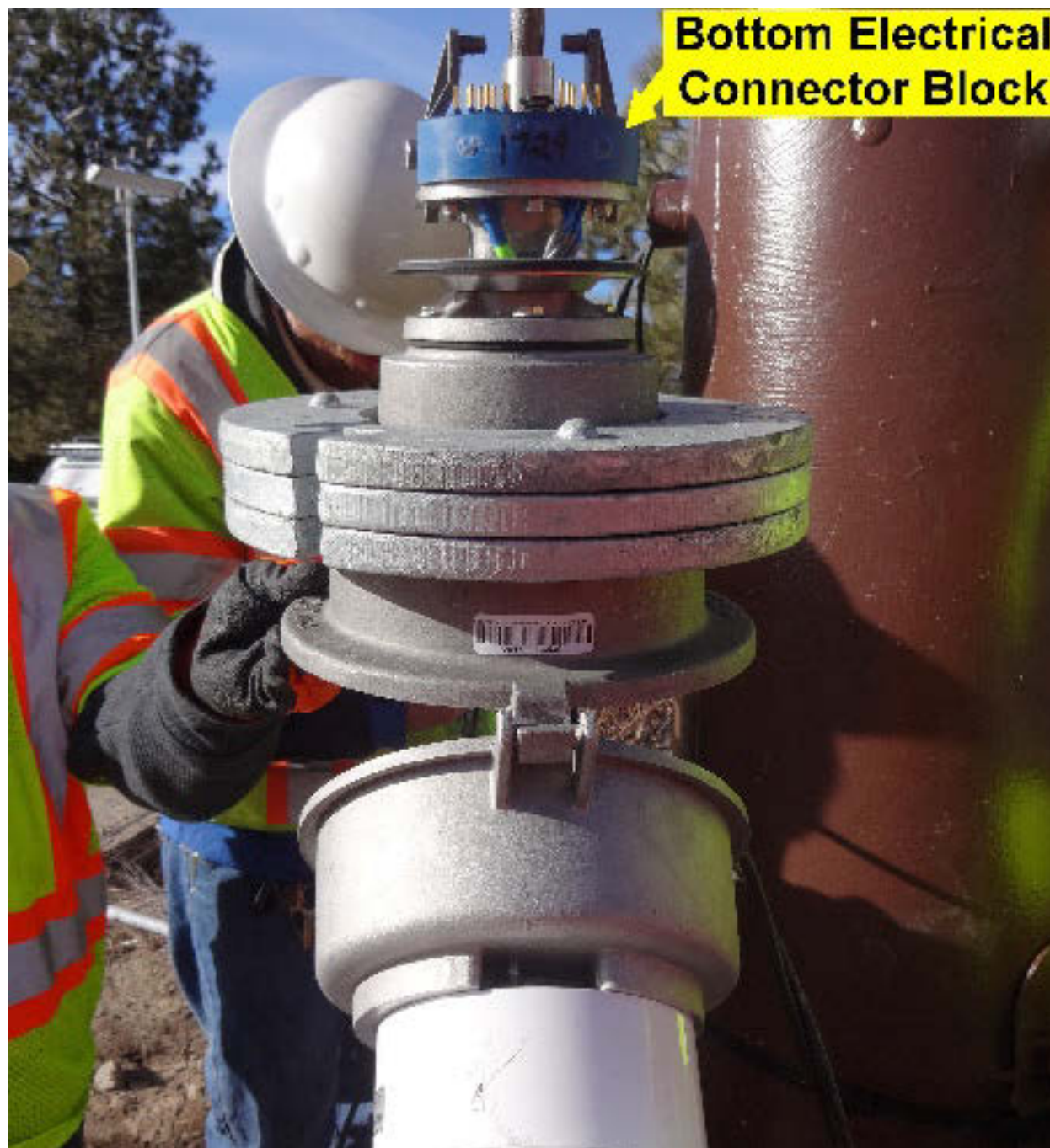
Figure 11. MG 2 E-Connector Installed
