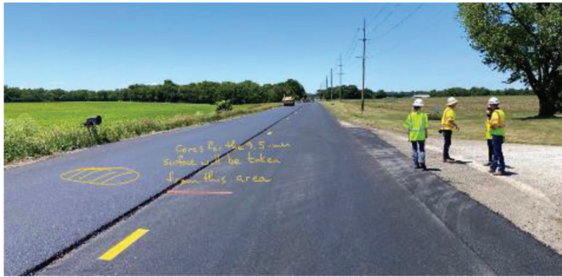
Figure 2.10 Cores for the 9.5-mm surface mixture taken at approximately Station 160+00, near the center of the project in the eastbound lane.
