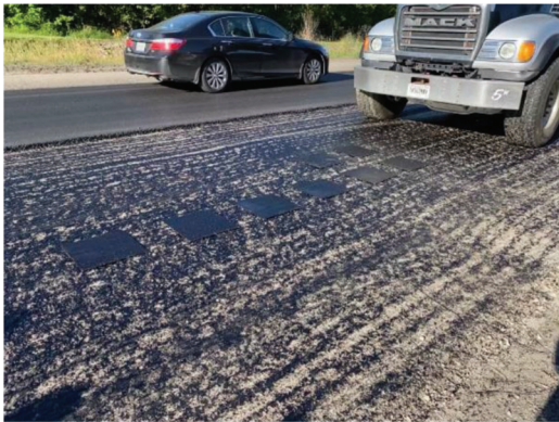
Figure 6.3 Layout of sample plates ahead of paver on U.S. 421.
