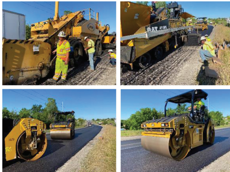
Figure 2.6 Construction equipment used on U.S. 421 project west of Delphi, IN.
