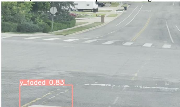
(g) Faded double yellow lane marking
