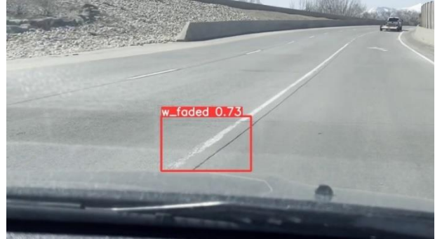
(b) Faded white lane marking
