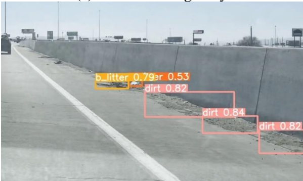
(c) Dirt and litter on the highway
