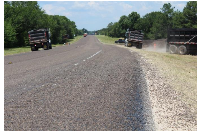
June 2020 (After the Construction)
