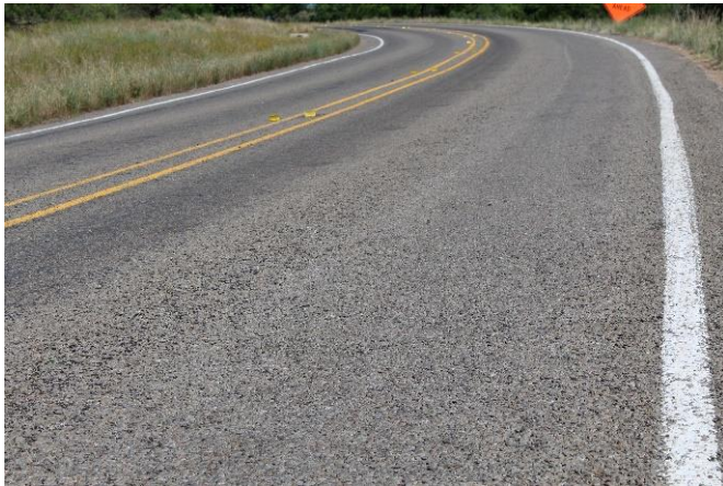
June 2020 (Before the Construction)
