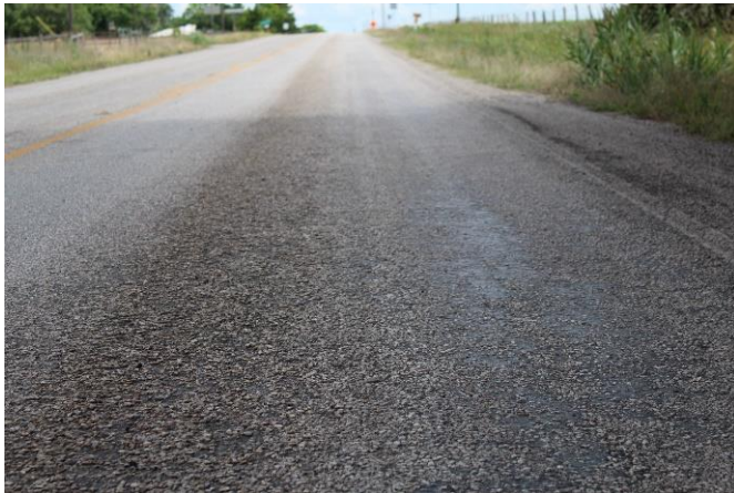
May 2020 (Before the Construction)
