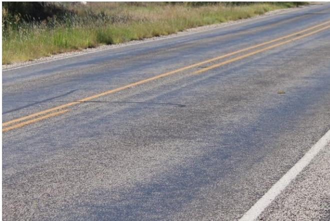
June 2018 (Before the Construction)
