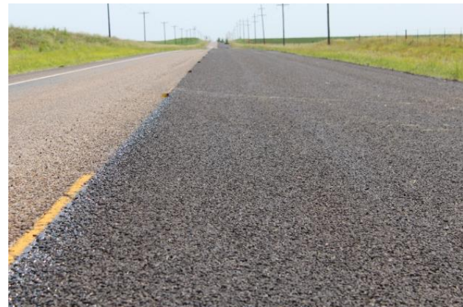
August 2018 (After the Construction)
