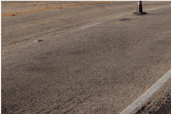
August 2018 (Before the Construction)
