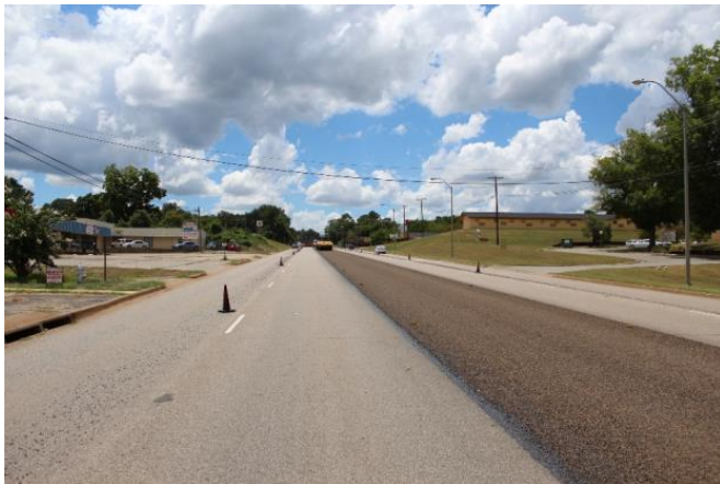
August 2018 (Before the Construction)
