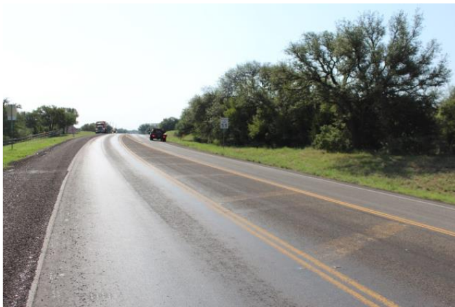
August 2018 (Before the Construction)
