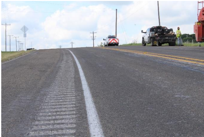
June 2020 (Before the Construction)
