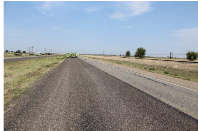
August 2018 (After the Construction)
