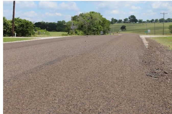
June 2020 (After the Construction)
