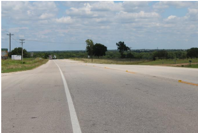
May 2020 (Before the Construction)
