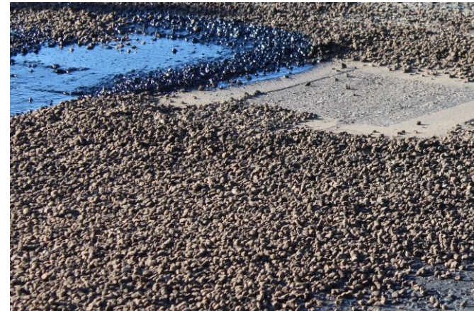
August 2018 (After the Construction)
