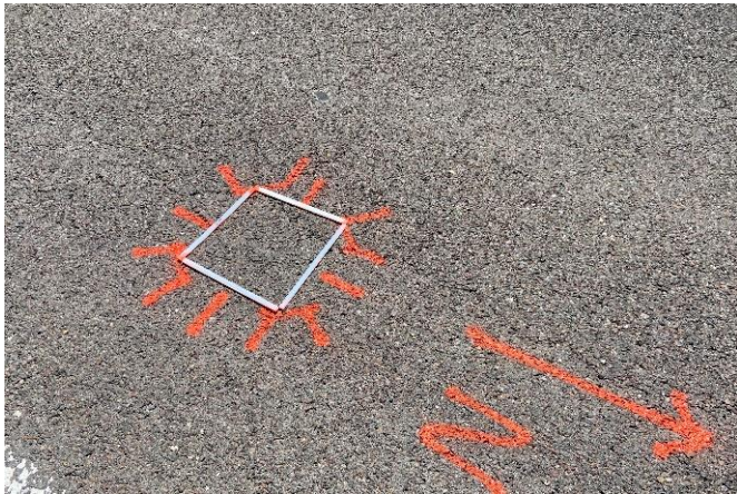
June 2020 (Before the Construction)
