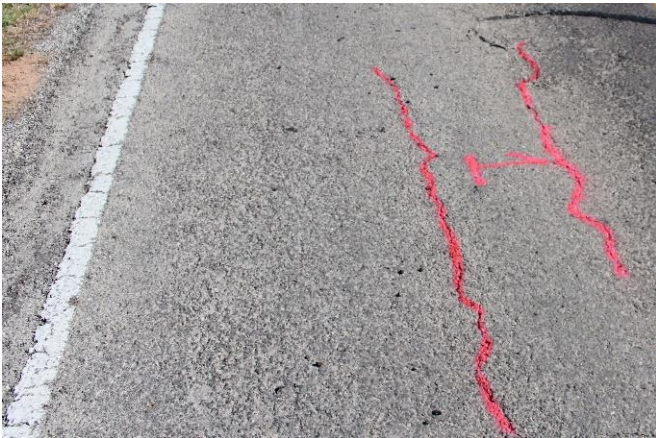
June 2018 (Before the Construction)
