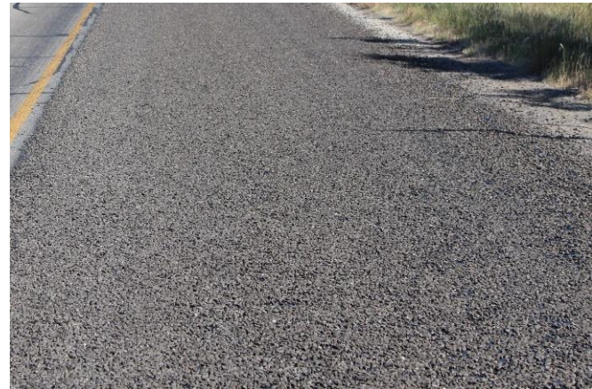
June 2018 (After the Construction)
