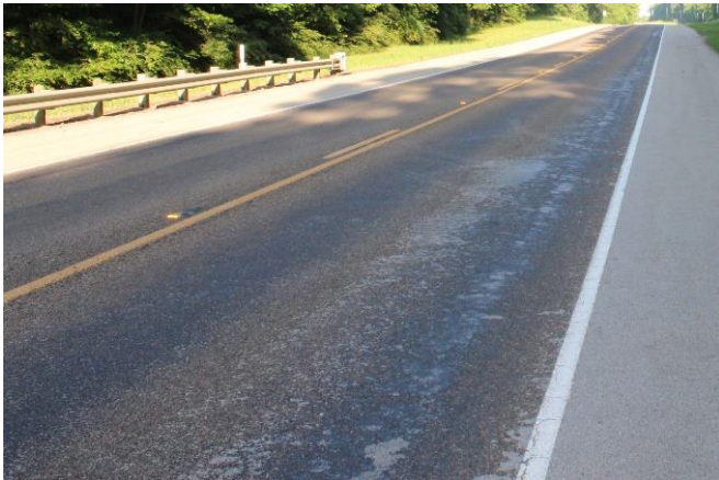
June 2018 (Before the Construction)
