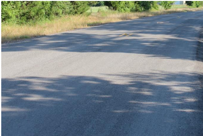
June 2018 (Before the Construction)
