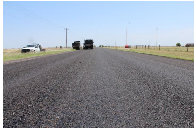
August 2018 (After the Construction)
