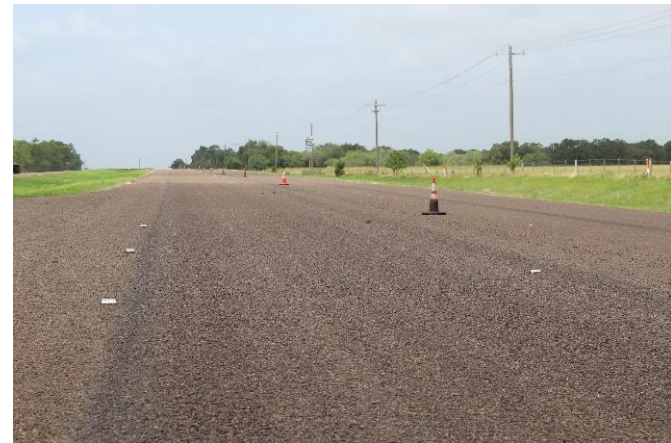
June 2020 (After the Construction)
