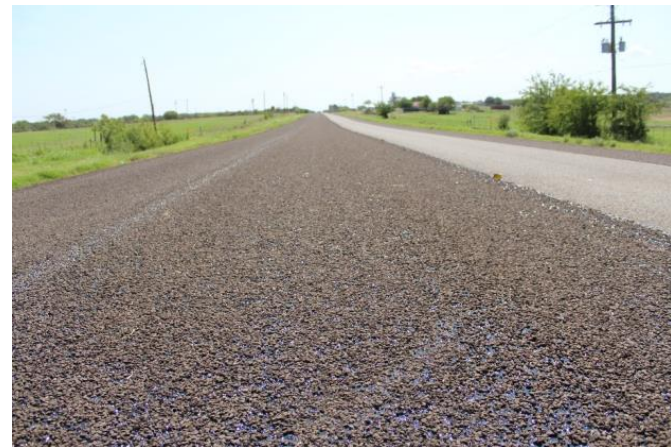
August 2018 (After the Construction)
