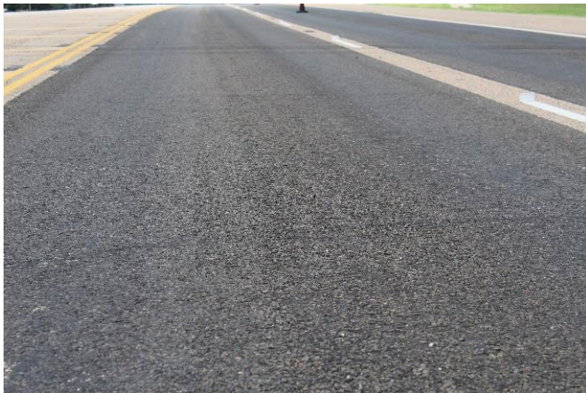
June 2020 (Before the Construction)
