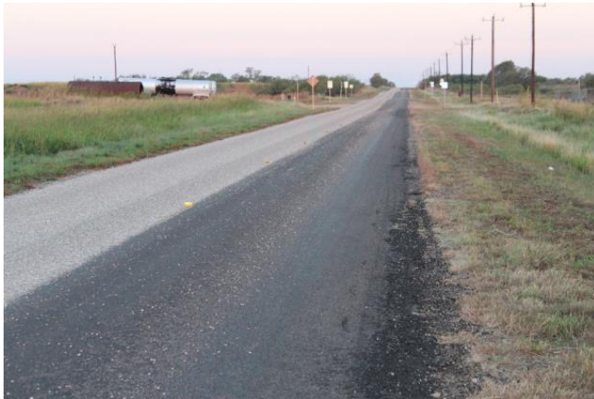
September 2018 (Before the Construction)
