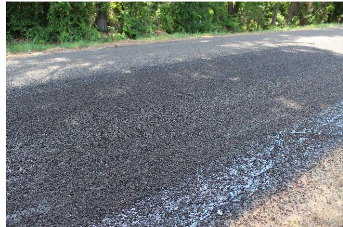
June 2018 (After the Construction)
