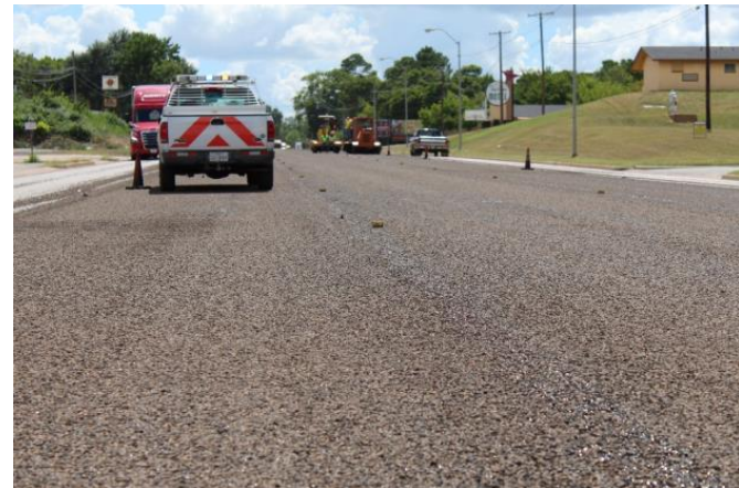
August 2018 (After the Construction)
