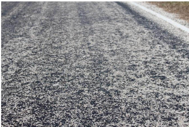
May 2020 (Before the Construction)
