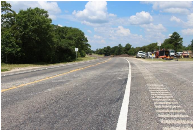
June 2020 (Before the Construction)
