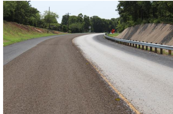
August 2018 (After the Construction)
