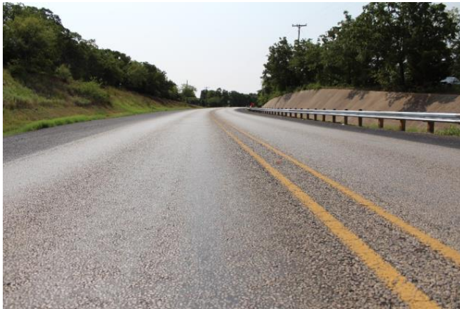
August 2018 (Before the Construction)
