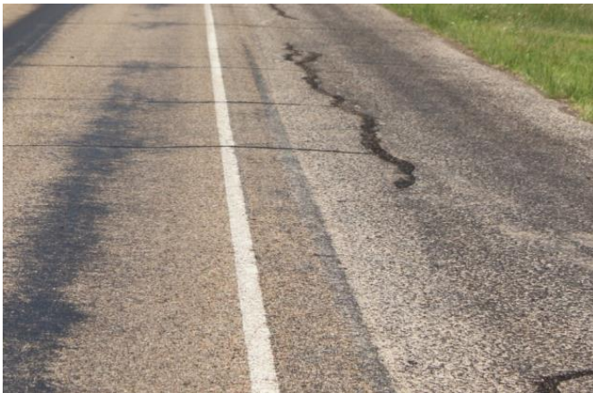
August 2018 (Before the Construction)
