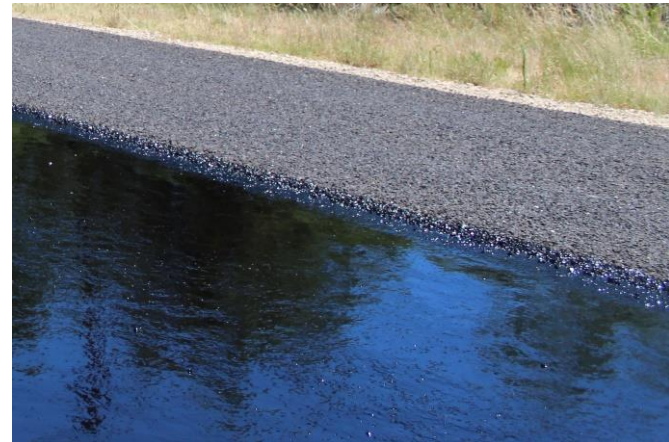
June 2018 (After the Construction)
