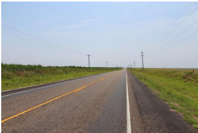
August 2018 (Before the Construction)
