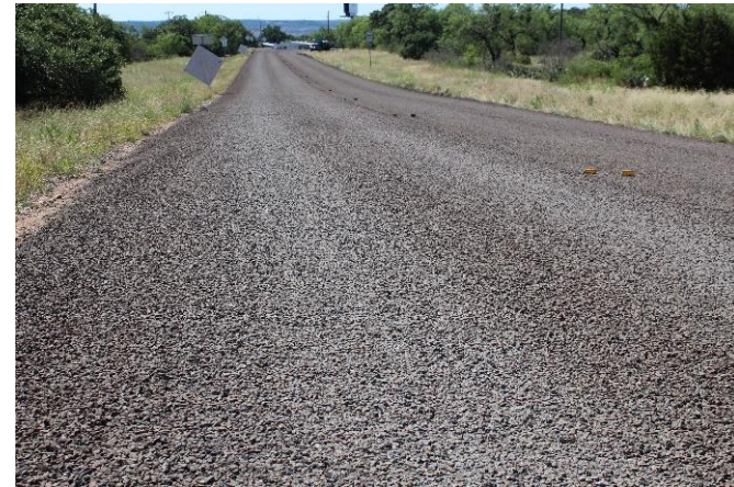
June 2020 (After the Construction)
