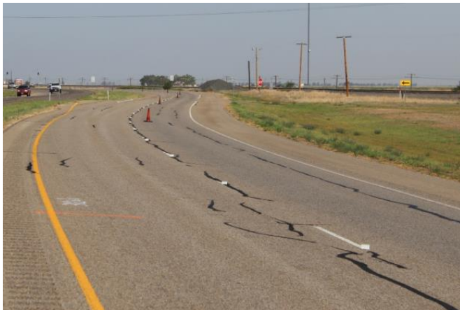
August 2018 (Before the Construction)
