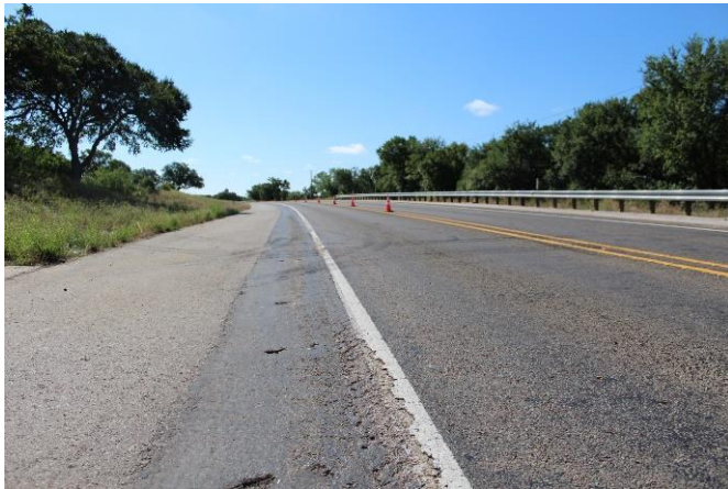
June 2020 (Before the Construction)
