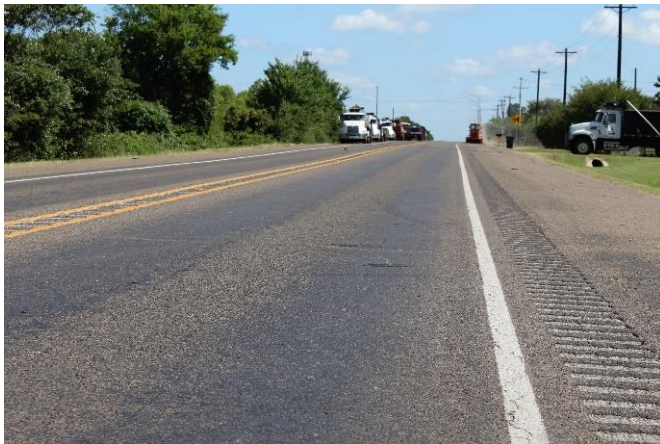
June 2020 (Before the Construction)
