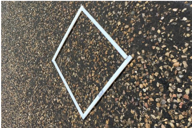
September 2020 (Before the Construction)
