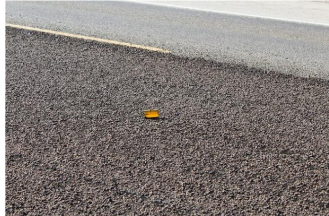
June 2018 (After the Construction)
