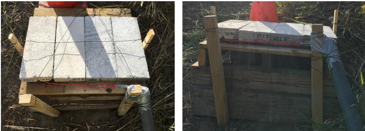
Figure 5.25. Mini slabs on the field site
