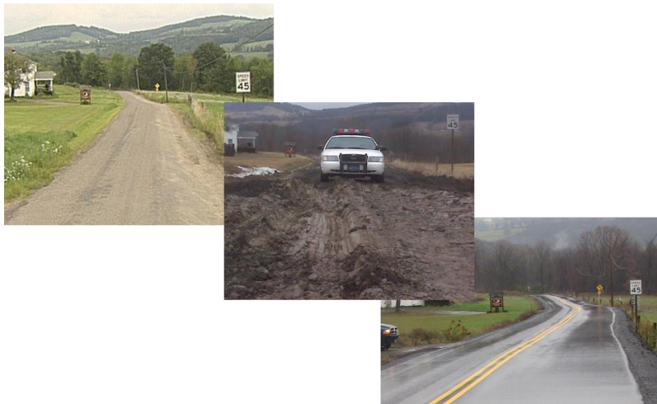
Figure 1. Roadway Impacts in Pennsylvania—Pavement to Mud and Then Restored.
