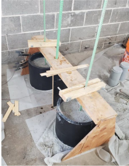
Pull-out test samples during casting
