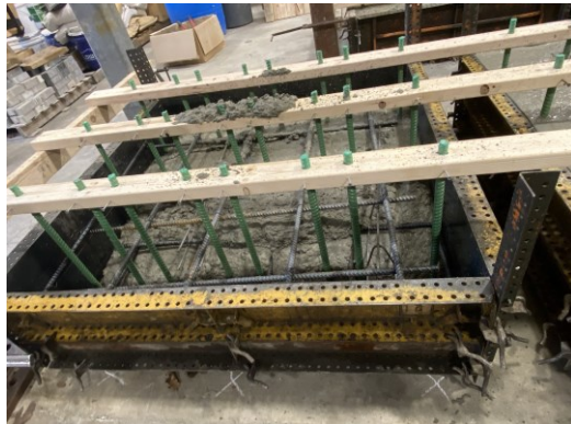
Filling the concrete slabs
