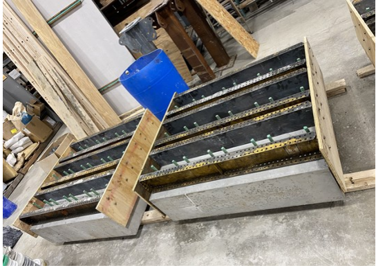
Building the formwork to cast the filling
