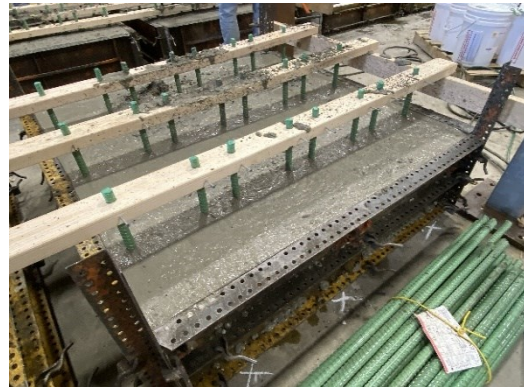
Concrete slabs after concrete placement
