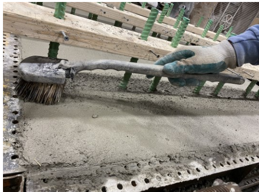
Finishing the surface of the concrete slabs
