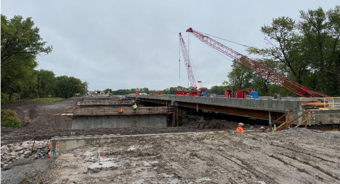
Superstructure of IA 1 bridge
