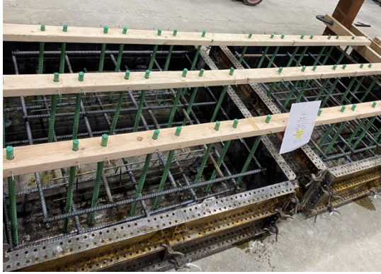
Vertically-fixed embedded rebars
