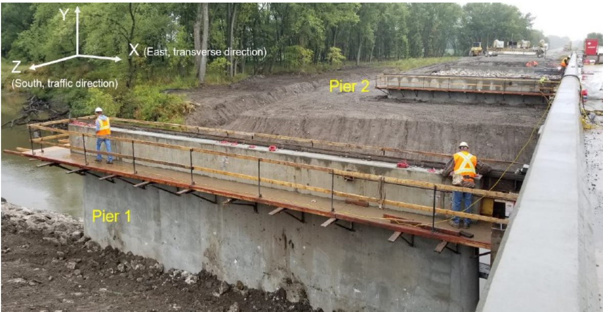
Substructure of IA 1 bridge with bridge orientation
