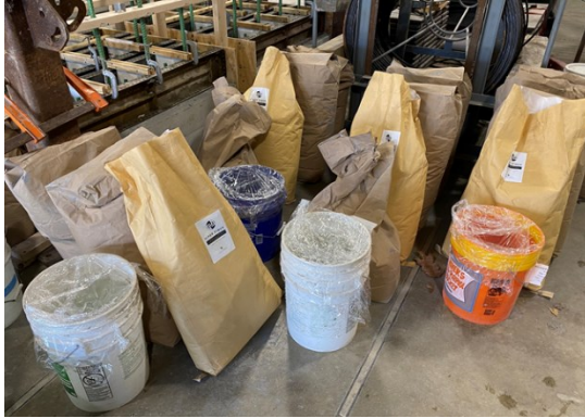
Preparing UHPC batches quantities
