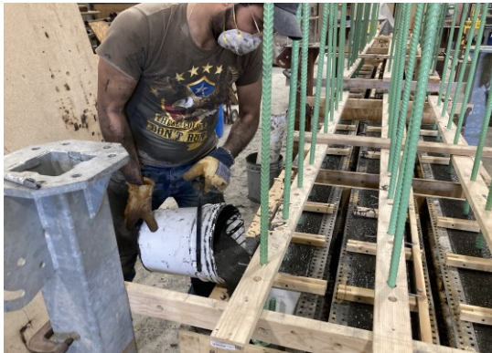
Pouring the UHPC in the forms
