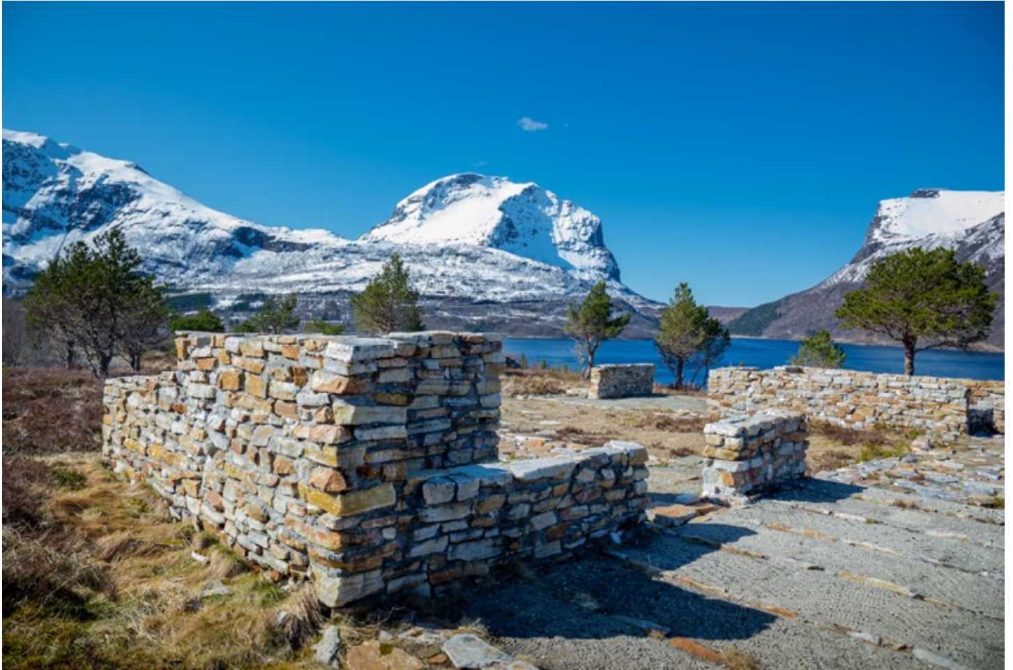
Figure 1. The Forgotten Town (1996), by Jan Håfström in collaboration with architect Johan Celsing. Sited near the village of Inndyr, Gildeskål, Norway. Photograph: Steinar Skaar & Knut Wold.
