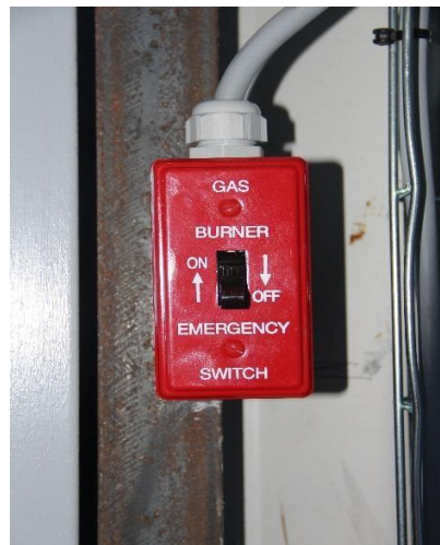
Figure 2.11: The emergency switch.
