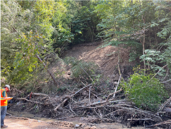
Figure 19. Photo of translational landslide along Hardshell Caney Road in Breathitt County, triggered by the July storms.
