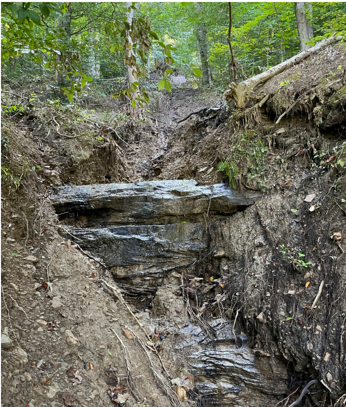
Figure 24. Narrow debris flow channel along KY 2446 in Perry County.
