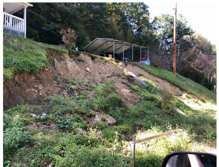
Figure 35. Landslide-damaged property in front of home off KY 484 in Perry County.
