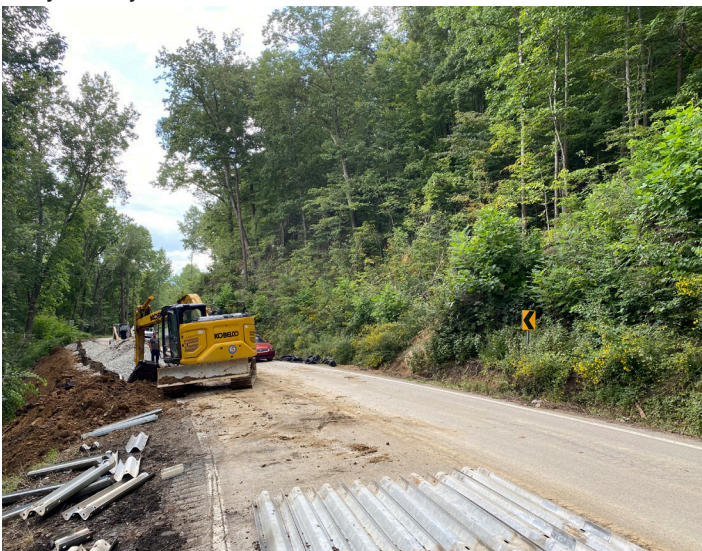
Figure 32. Road stabilization work after a landslide damaged KY 28 in Perry County.
