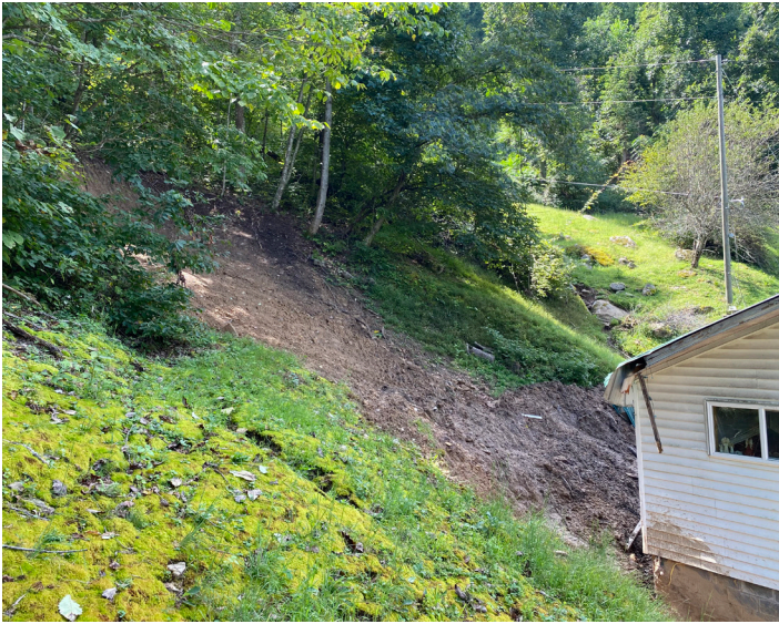
Figure 18. Photo of a translational landslide behind home, triggered by the July storms.
