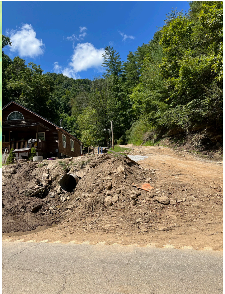
Figure 42. Field-checked debris flow from Figure 41 identified in HazMapper. The debris fan at the mouth of the catchment (marked by the star on the rdNDVI map) threatened the home and was deposited along KY 550 in Knott County.
