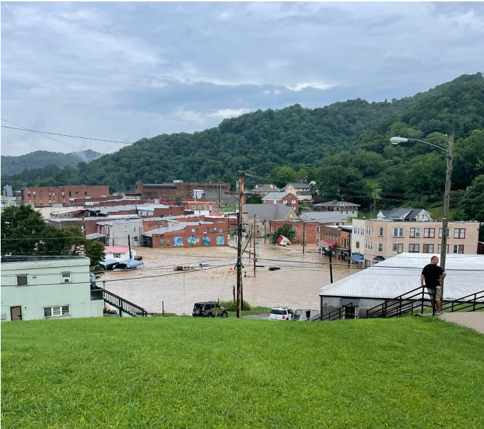
Figure 2. "Severe flash flooding caused extensive damage in downtown Whitesburg, KY." (NOAA National Weather Service, 2022).
