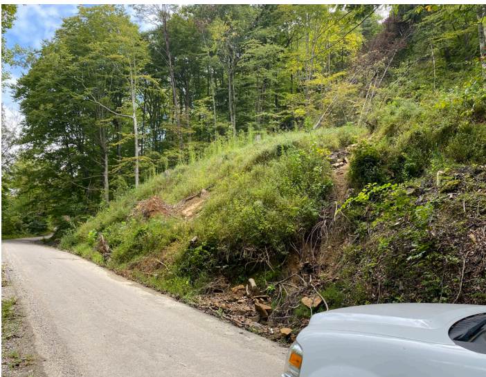
Figure 22. Slump observed off KY 28 in Perry County. Note tilted trees in the upper part of the slide.
