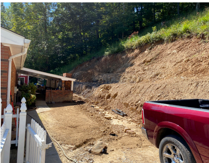
Figure 34. Translational landslide behind home near KY 451 in Perry County.
