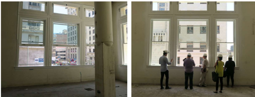
Figure 4-7 window film reducing heat gain applied to listed building in Los Angeles. Left – blue tint was not accepted by historic preservation committee. Right – colorless film was approved (Adapted from Boote 2018)
