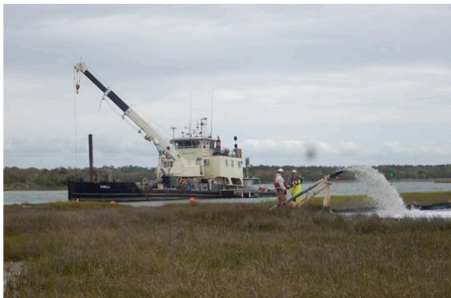
Fig. 7. Application of dredged sediment from the Atlantic Intracoastal Waterway to marsh pond. The filled pond was subsequently planted with Spartina alterniflora , maintaining the integrity of the marsh platform adjacent to the navigation channel.
