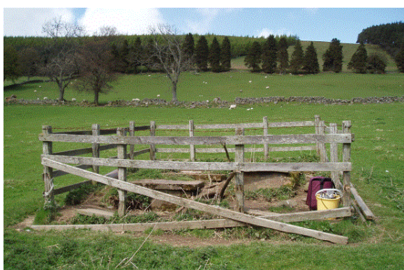
Figure 10 Two different springs on the monitoring network. Even where sources are fenced, the fence is often in disrepair. Spring boxes are generally brick lined with a cement screed, and are best sampled from an inflow.
