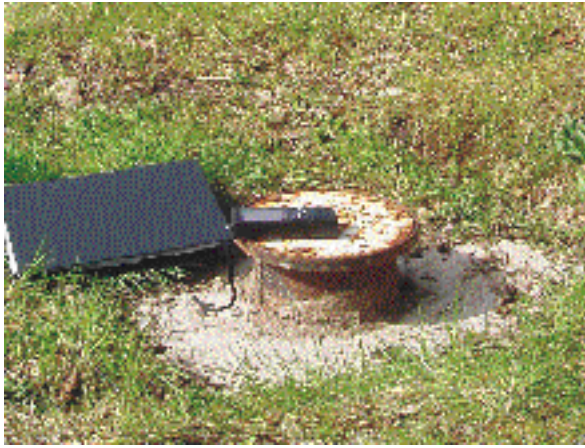
Figure 14 A purpose drilled observation borehole (left) and the headworks of an effectively constructed pumping borehole (right).
