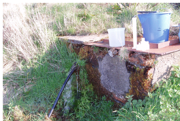
Figure 10 Two different springs on the monitoring network. Even where sources are fenced, the fence is often in disrepair. Spring boxes are generally brick lined with a cement screed, and are best sampled from an inflow.
