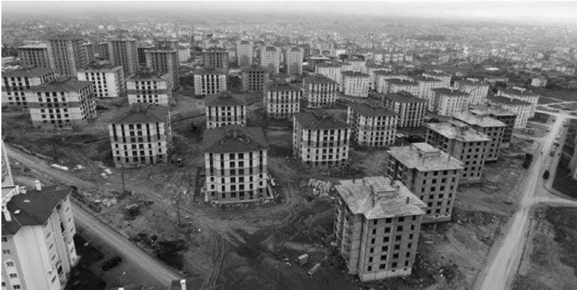
Image 3.5 The construction of the new TOKI apartments.
