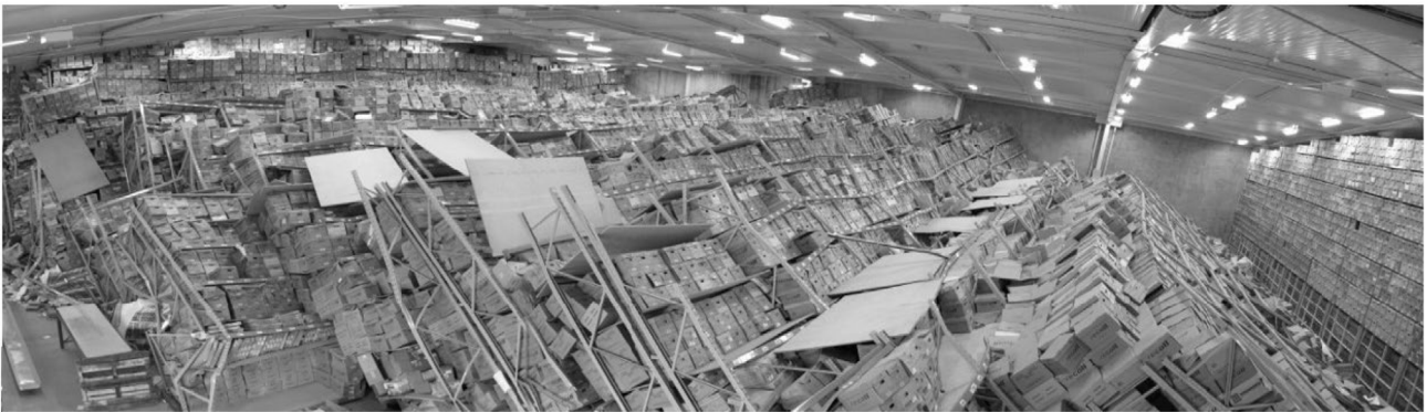
(c) Progressive collapse of the whole facility
