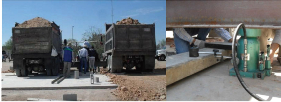
FIGURE 5: Field mounting for slab deformation.
