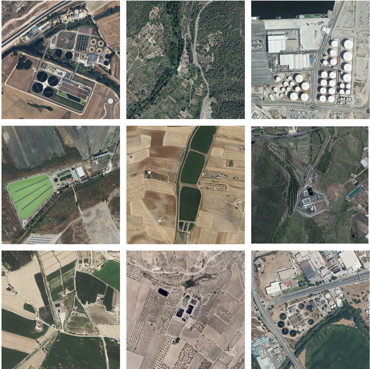
Figure A1: WWTP infrastructures vary wildly in size and morphology, depending on the underlying technology and the type of treatment they perform. However, they generally stand out for the circular or rectangular structures of settlers, tanks, and trickling filters. These very high-resolution orthophotos from the Spanish National Geographic Institute (IGN) are displayed at the same scale to make their differences more evident.
