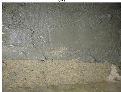
(b)shotcreting upper parts
