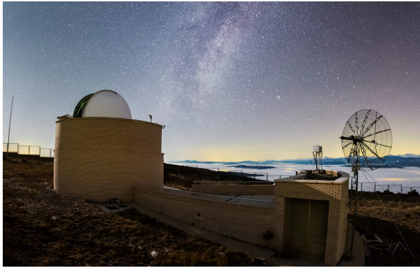
Figure D.1: Montsec Ground Segment. Image credit: Kike Herrero (IEEC)
