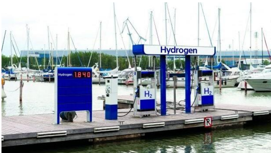
Figure 21. Hydrogen fuelling station
