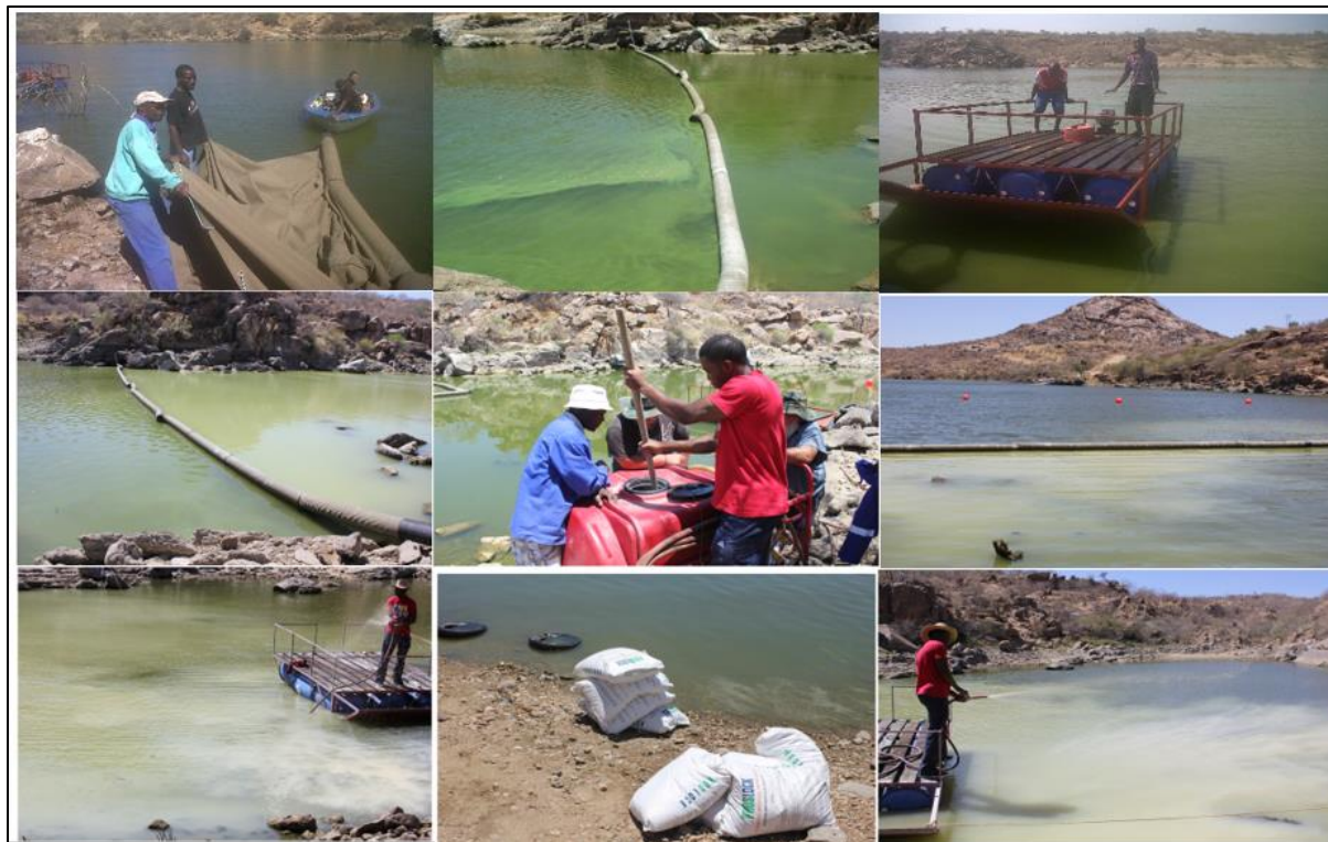
Figure 6.2. Pictures of the application of Phoslock as a phytoplankton control measure in the SWP Dam from 14 November 2012 to 16 November 2012 for a period of 3 days.
