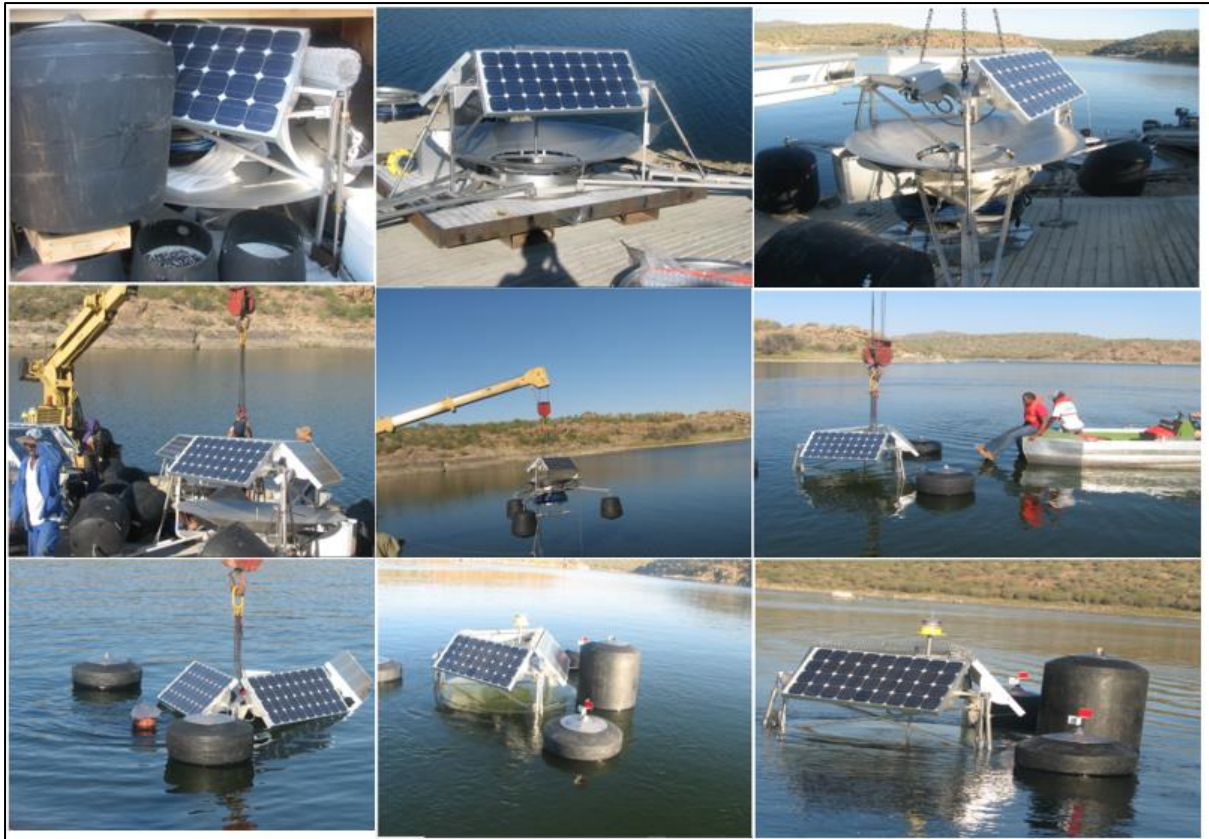
Figure 6.3. Pictures of Solar Powered Circulation installation as a phytoplankton.
