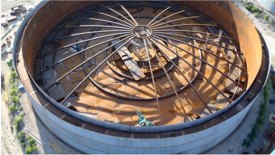
Figure 2.11. Double-wall external FRT [111]
