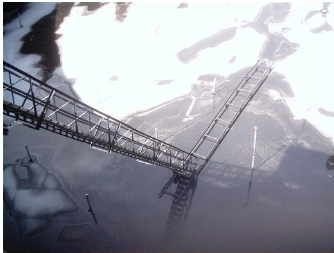
Figure 7.8. Oil spills on the roof
