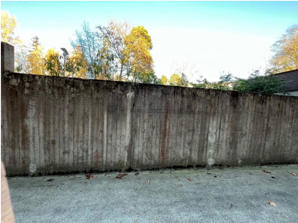
Figure 36- Reinforced Cocnrete Retaining Wall in Aalto University
