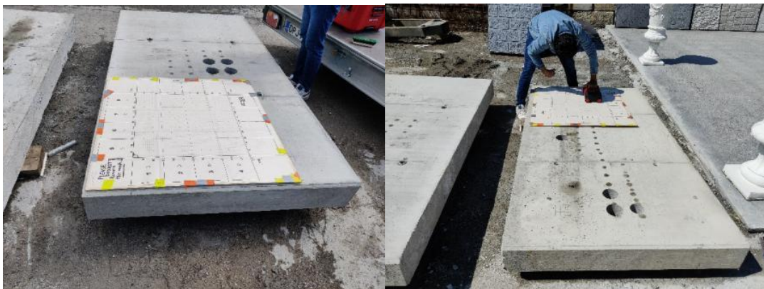
Figure 39- GPR scanning of Precats Reinforced Cocncrete Slabs
