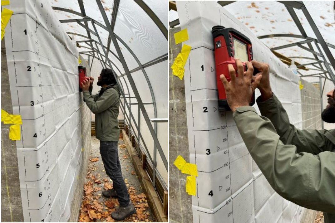
Figure 32- GPR Scanning of Side-B
