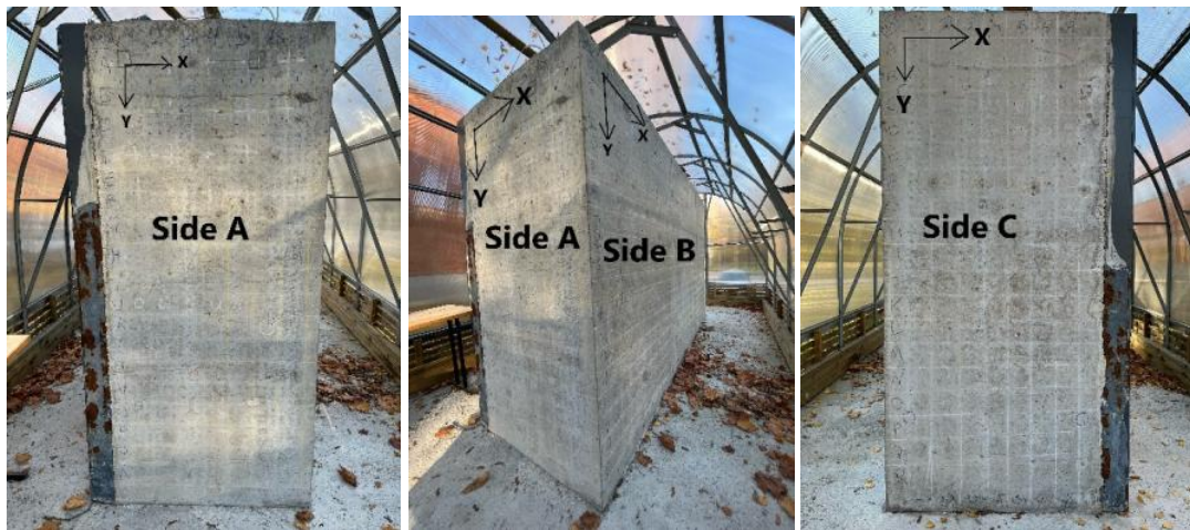
Figure 29- Three Sides of Concrete Mockup Wall
