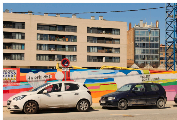
Fig. 4. Construction works next to Cristóbal de Moura Street with graffitis that read “no offices” and “we want green spaces” (Source: Authors, 2021).
