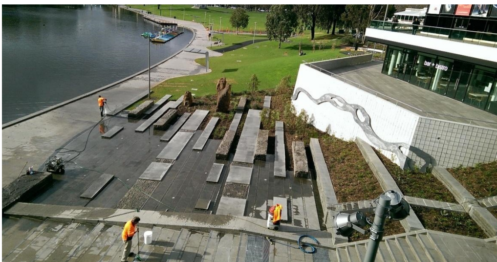
Figure 9-42: Maintenance activities in (Stella Bowen Park/Tarntanya Wama, Park 26). (Photo by author 2014)
