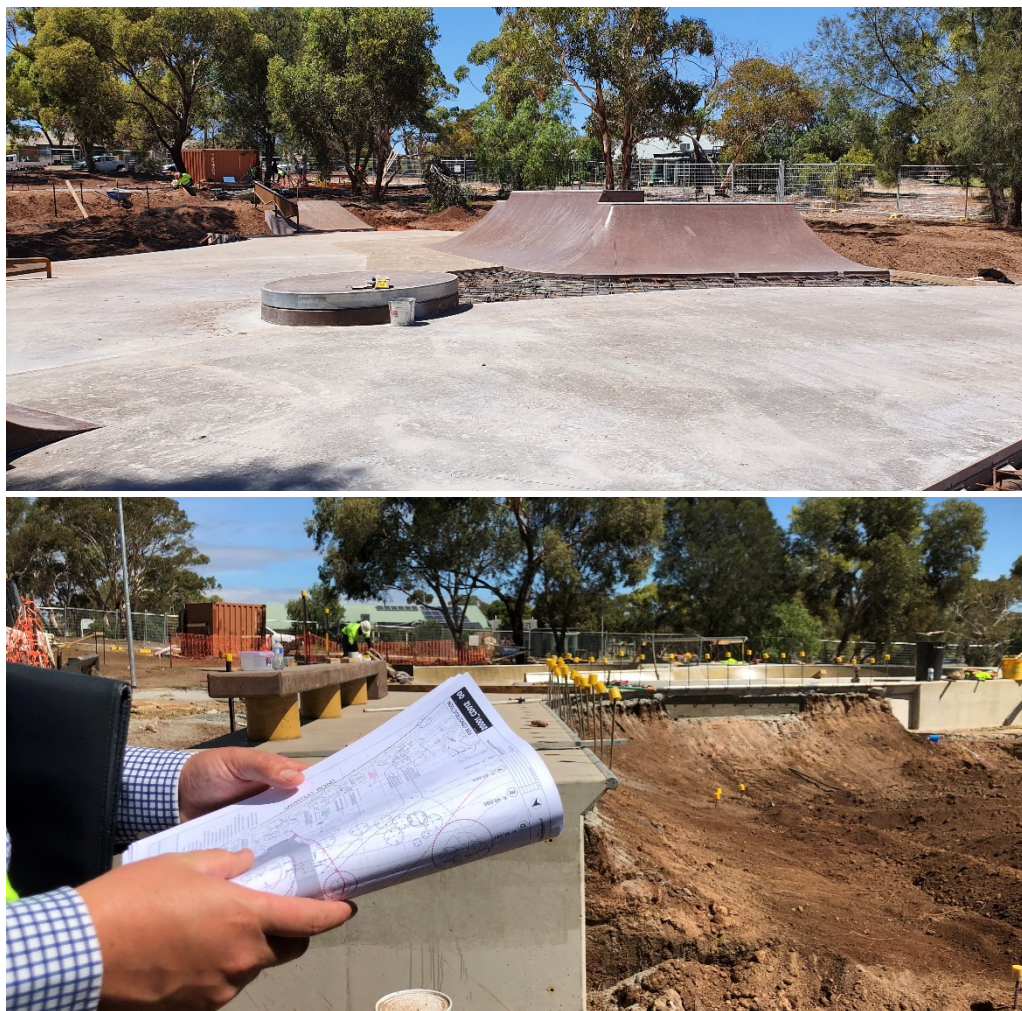
Figure 10-4: Morton Road Skate Park in construction. (Photo by author 2021)
