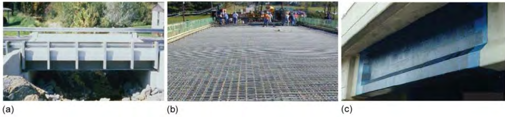
Figure 2.1. Examples of the use of FRP materials as: (a) building complete structure, (b) reinforcing method and (c) strengthening method [4].
