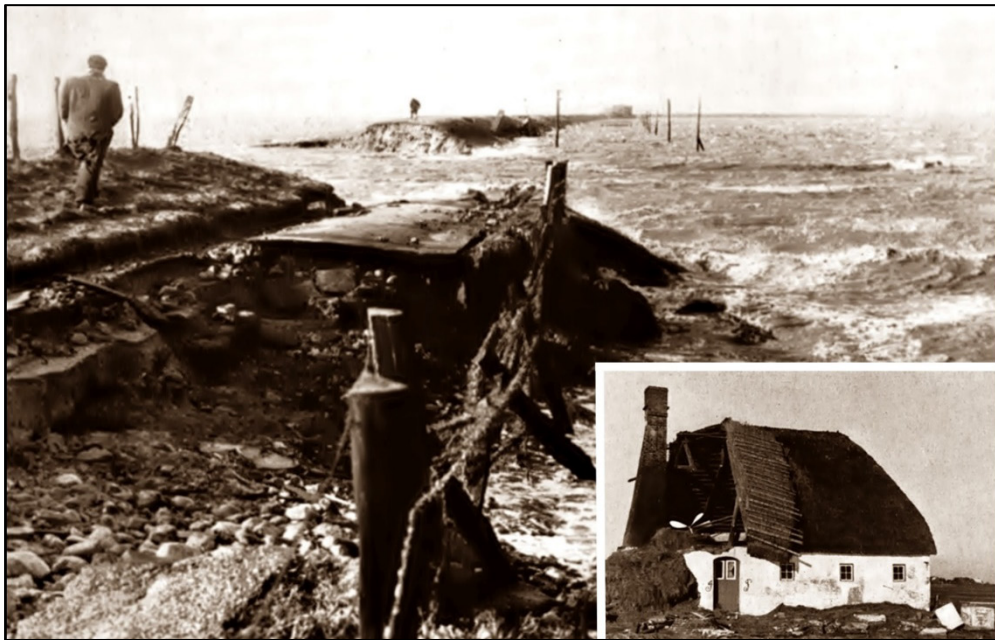
Figure 1: Dike breach in the polder Dockkoog near Husum after the 1962 storm surge (source: MELFF 1962). The inset shows a destroyed house on the Hallig Langeneß (source: Wohlenberg 1962).
