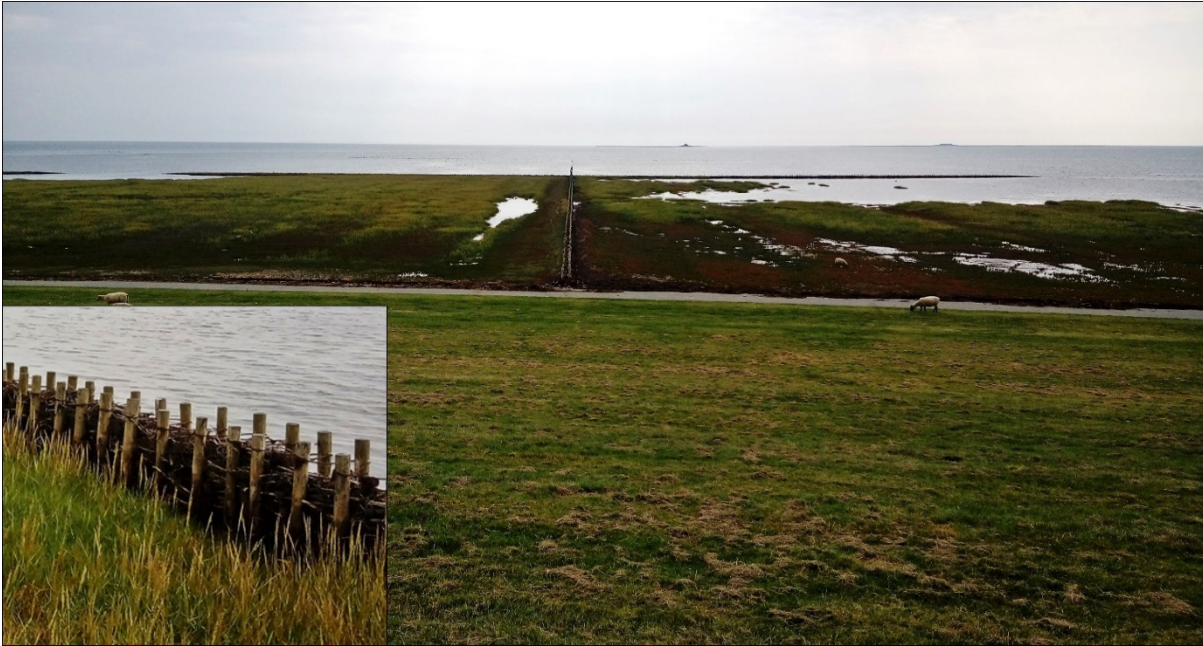
Figure 7: Brushwood groin fields in front of a state dike in Schleswig-Holstein. The inset shows a close-up of a brushwood groin. Note the newly developed vegetation cover behind the groin. (photos: Jacobus Hofstede).
