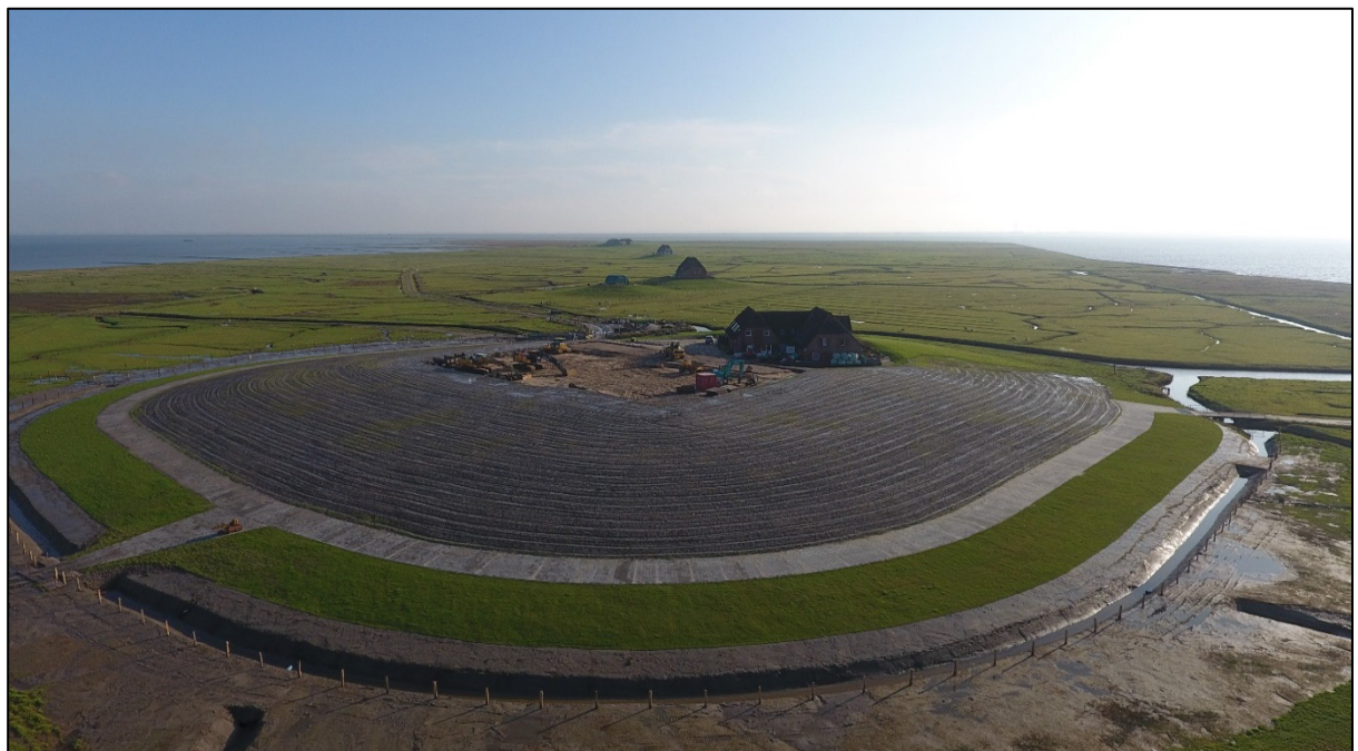
Figure 14: Plateau-reinforcement on the Hallig Nordstrandischmoor. The height difference among the existing mound with the house and the new plateau is about 1.5 m. (©: Thore Siefert).
