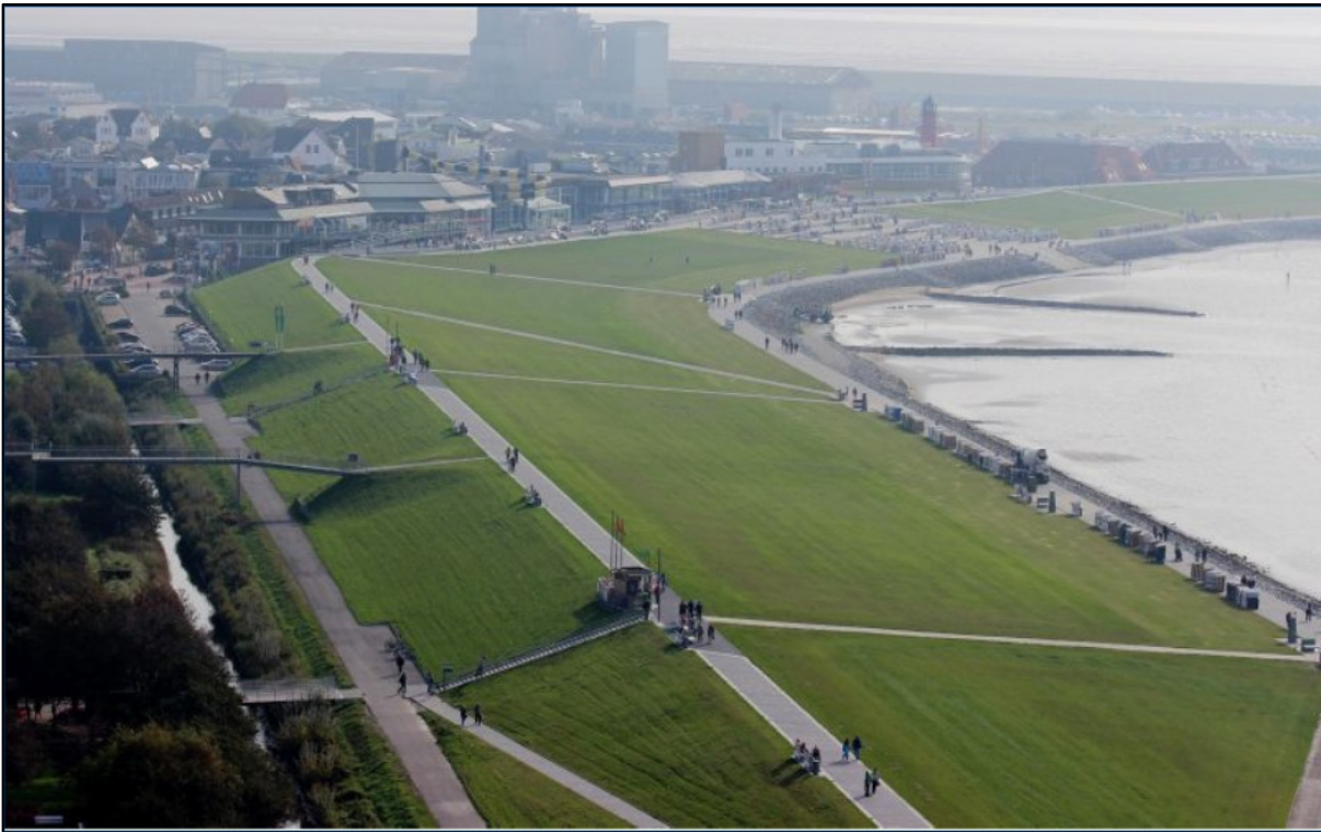
Figure 12: Strengthened dike in front of the tourist resort Büsum with a flat outer dike slope, a broad dike crest and a safety allowance of 0.5 m (Photo: LKN.SH).
