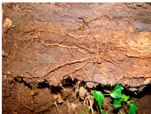
Figure 3. Crib wall logs in an advanced deterioration state (Artía river, Irún, Spain). Plant roots are occupying the space previously filled by tree logs while adsorbing nutrients coming from the decomposed wood. Source: Guillermo Tardio.
