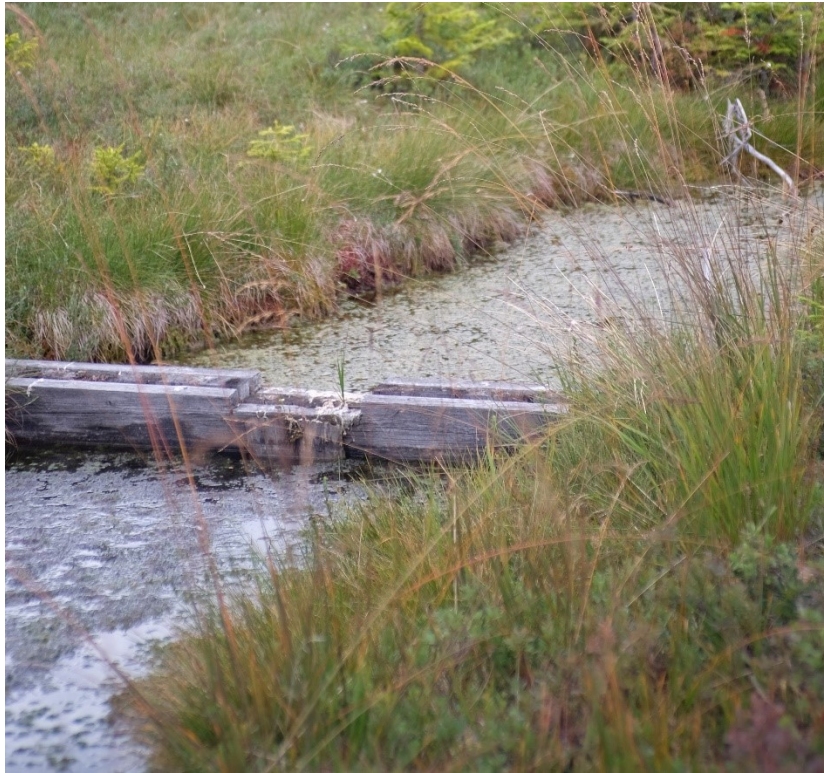
Figure 2: A wooden dam in Šumava National Park Photo: A. Kevešová, 2022
