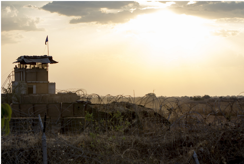
Figure 3: Fortifications on one of the barriers protecting the POC site, manned by UNMISS troops from the Indian Battalion (INDIABATT)
