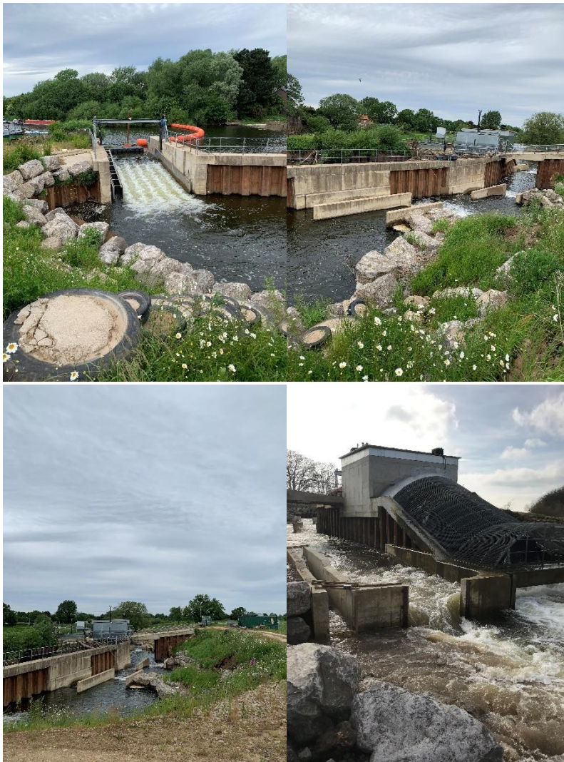
Figure 3.4. Different views of the co-located fish pass located adjacent to the hydropower turbine at Linton-on-Ouse Weir, opened 7 March 2019, from the upstream end of the pass (top, left) to the downstream end (bottom, right).
