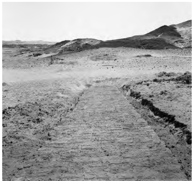
Figure 4.09 Wall [10-Y-12]. View down slope to southwest of tower A into area of deep sand.
