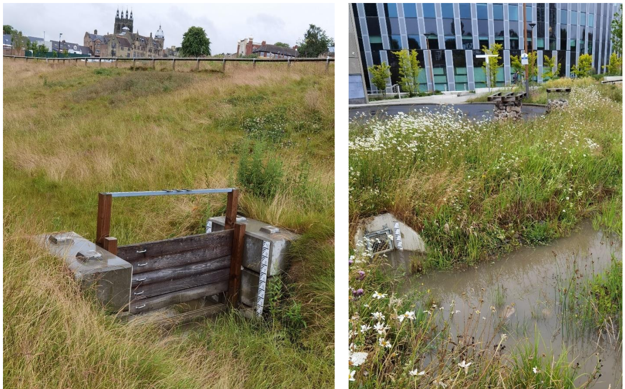
Figure 2. 5 Photos of Extreme Event Swale -a sustainable drainage system included in the National Green Infrastructure Facility of Newcastle University. (Image Jiaqian Wang)
